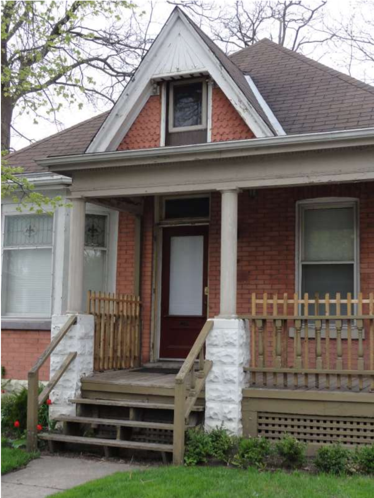
Image 5: Detailed view of front dormer (east) at 104 Wharncliffe Road North (May 11, 2018)
