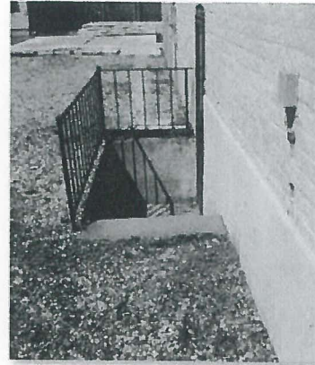
Image 2: Basement Stair at Grade (West Side of House)
