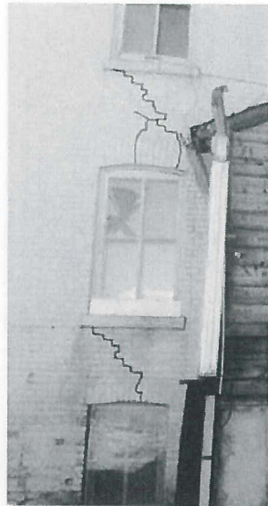
Image 6: Rear Brick Wall
