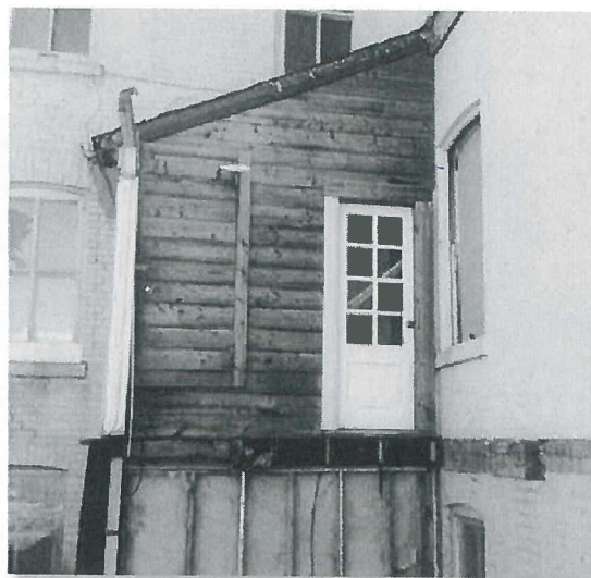
Image 9: Exposed wood framing (at Rear)
