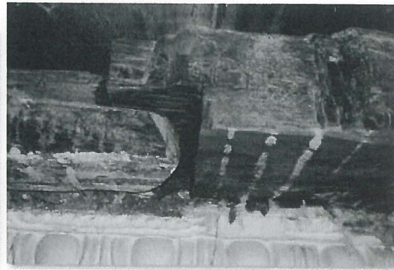
Image 15: Connection of Double Cantilever Joists At front of house
