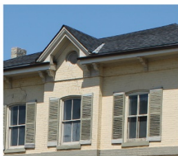
6. Shallow pitched hipped roof with gable roof emphasizing middle bay
