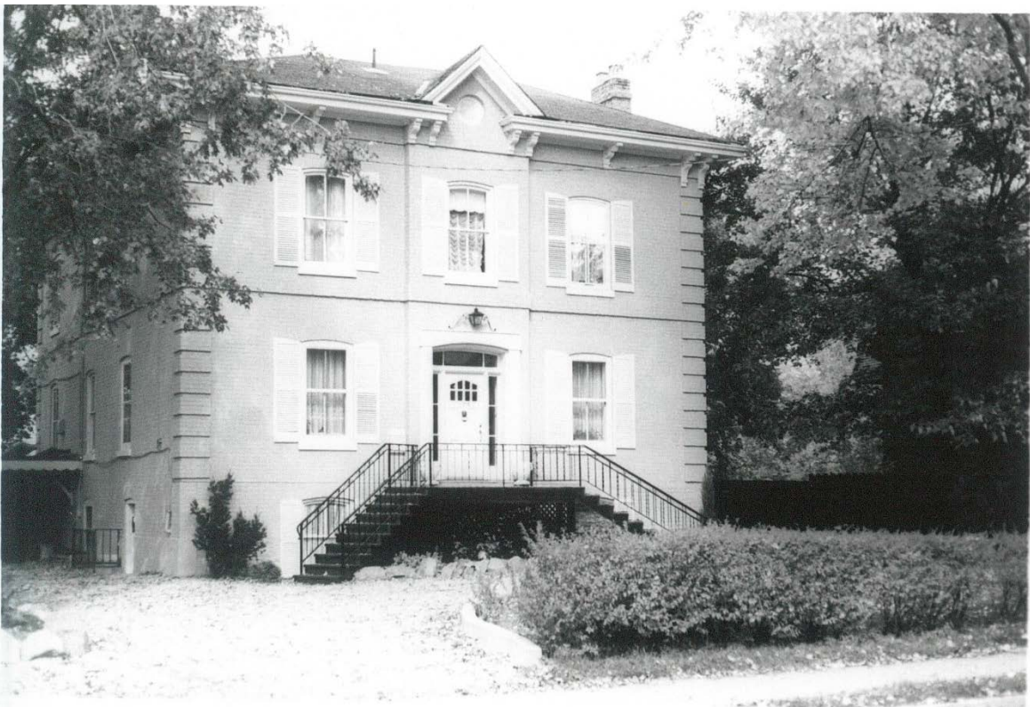
Image 2: Photograph of the property at 172 Central Avenue in 1977 by John Piccur.
