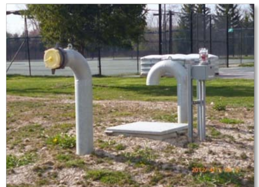
Figure 5: Underground Tank with Vent and Access
