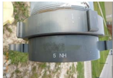
Figure 2: Swivel Fitting w/ 5" NH Female Swivel
