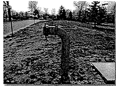
Figure 1: Drafting Port Side View - 90 Deg Elbow
