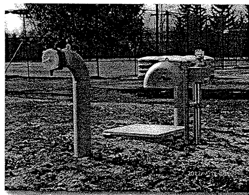
Figure 5: Underground Tank with Vent and Access
