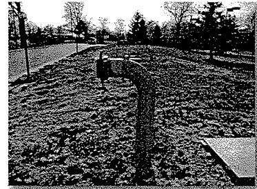
Figure 1: Drafting Port Side View - 90 Deg Elbow
