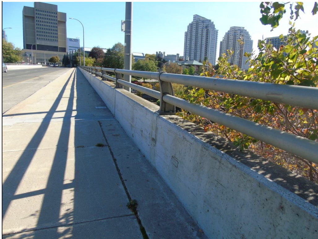
Image 21: Curb, parapet, and railing system located on The Queen's Bridge
