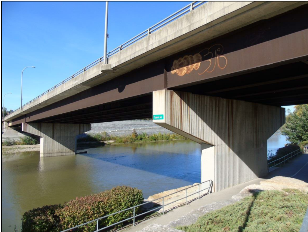
Image 11: View showing south side of The Queen's Bridge, showing piers, welded steel girders, and the TVP trail on the east side of the river
