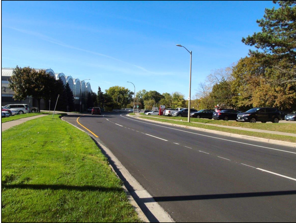
Image 16: Queens Avenue, showing curvature of the road at east approach to the bridge
