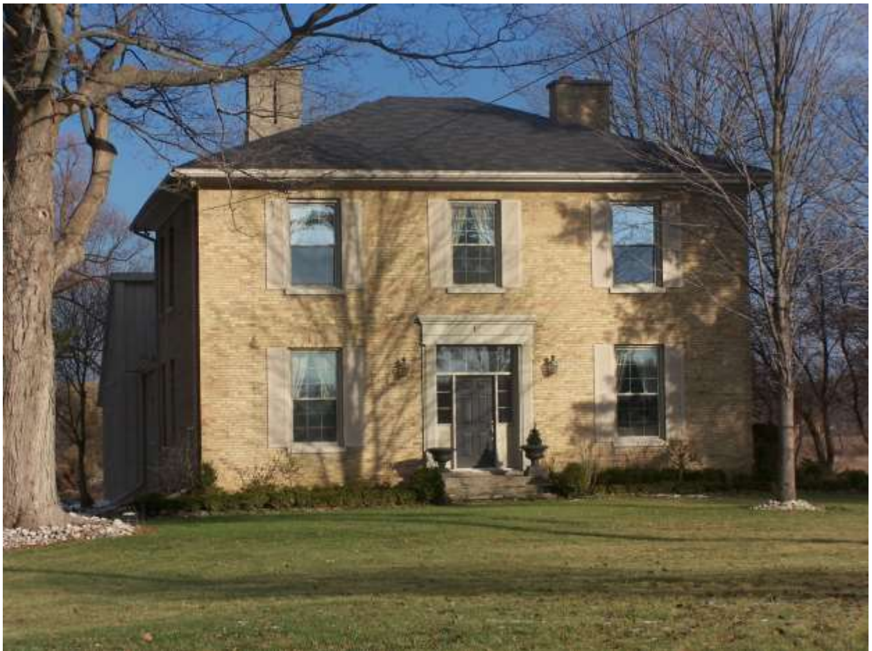
Image 6: Detail of the main (west) façade of the building located at 2096 Wonderland Road North (November 2007).
