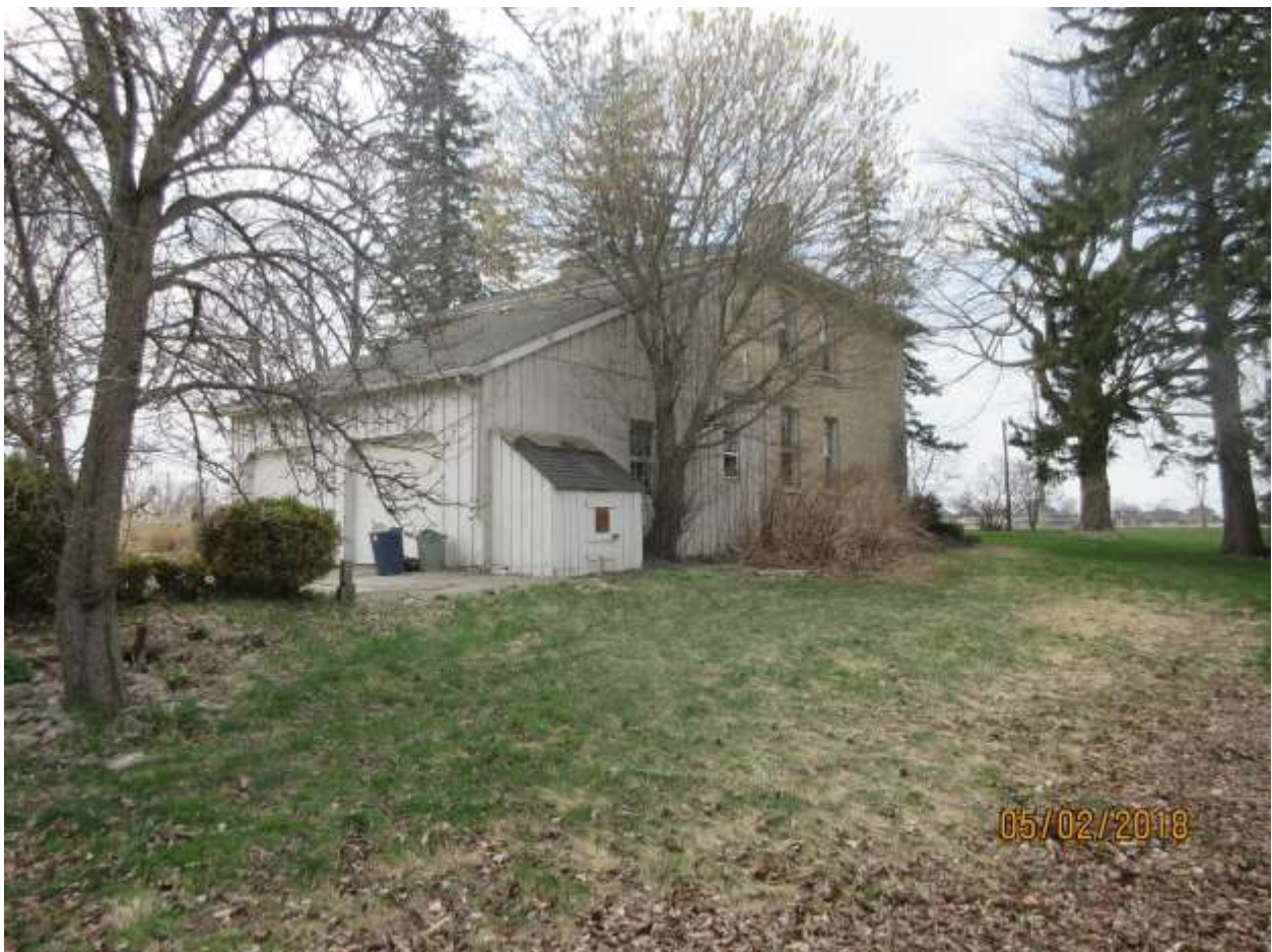
Image 10: View of the north façade of the building located at 2096 Wonderland Road North. Note: the wood board and batten clad addition to the original brick structure.
