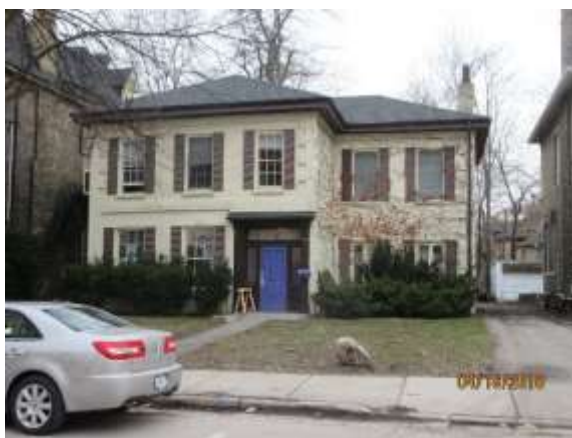
Image 15: Property at 130 Kent Street, built in 1863. Note the side hall plan of the building, painted brick, and asymmetrical massing.
