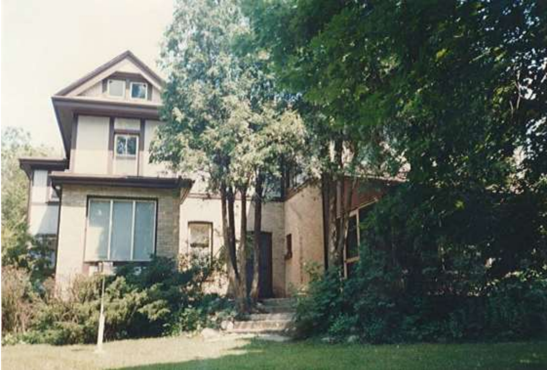
Image 1: Main (west) façade of the house at 2154 Richmond Street (courtesy of Middlesex Centre Archives, London Township Local Architectural Conservation Advisory Committee files, 1990).
