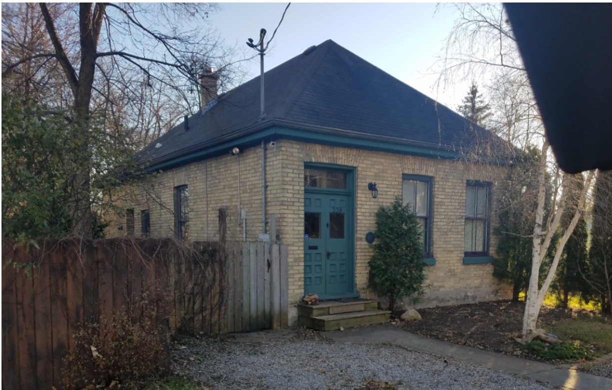
8. 239 Hill Street looking south
