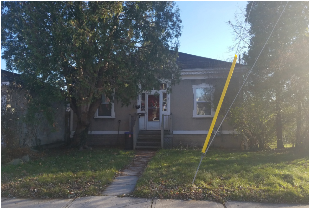
6. 267 Hill Street looking south
