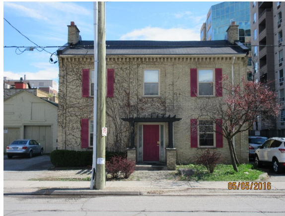
Image 16: Property at 177 Kent Street, built circa 1860. Note the urban context of this property, which translates into projecting firewalls at the gable ends of the building.
