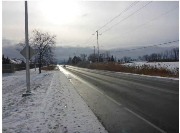
Plate 3: Wonderland Road north looking South from subject property
