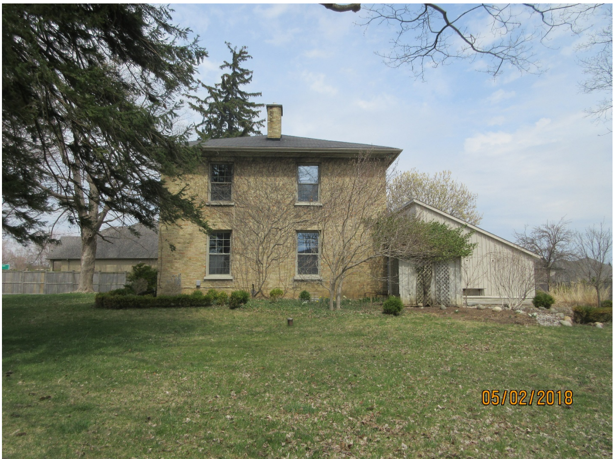
Image 8: South façade of the building located at 2096 Wonderland Road North. Note the rear addition.
