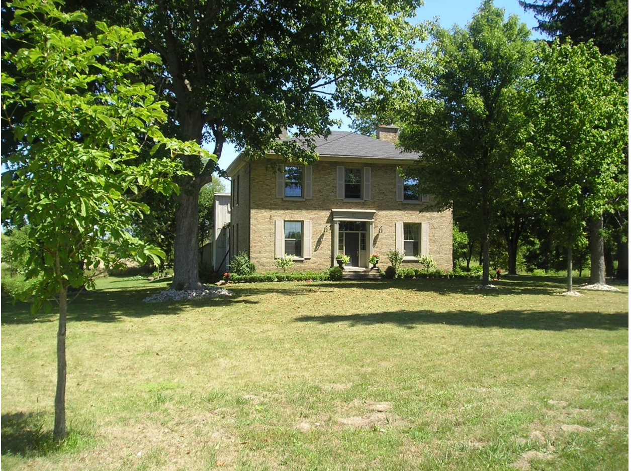
Image 5: View of the main (west) façade of the building located at 2096 Wonderland Road North on August 14, 2007.
