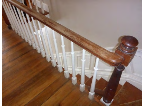
Plate 24: Staircase from 2 nd floor
