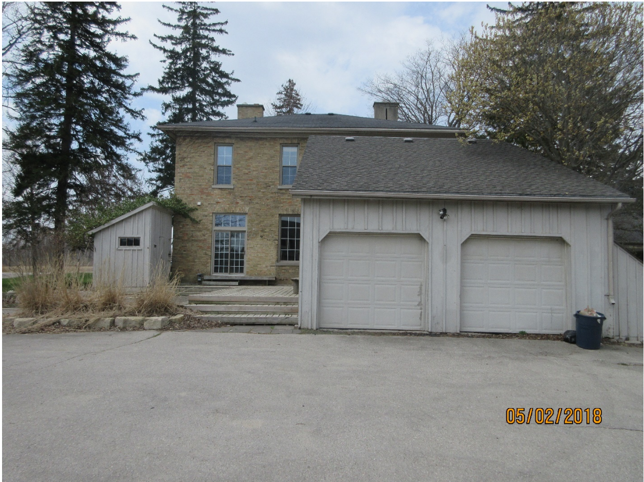
Image 9: View of the rear facade of the building located at 2096 Wonderland Road North.
