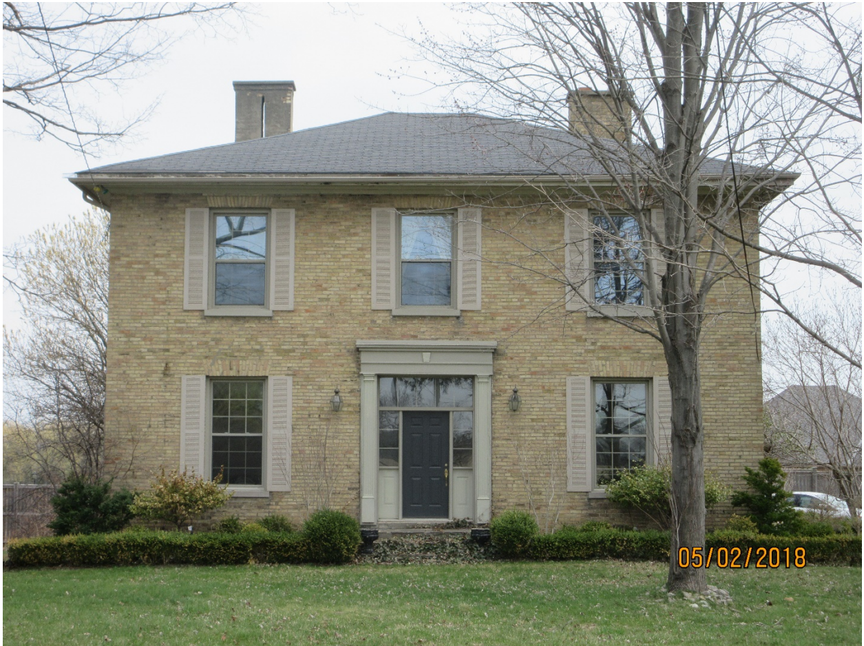
Image 7: Main (west) façade of the building located at 2096 Wonderland Road North.
