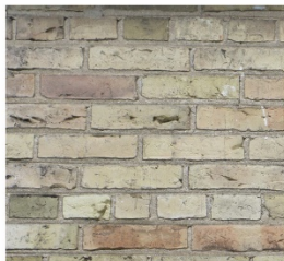
5. Buff brick construction
