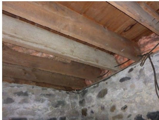
Plate 32: Basement with joists and foundation
