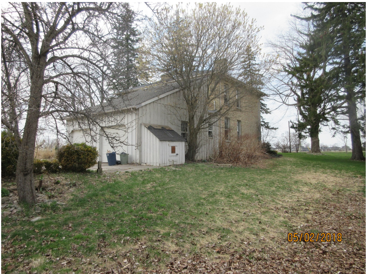
Image 10: View of the north façade of the building located at 2096 Wonderland Road North. Note: the wood board and batten clad addition to the original brick structure.
