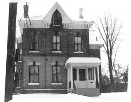
View of front (north) façade of dwelling showing past entrance enclosure and steps, note discoloration line indicating possible previous porch extending across the façade (precise date of photo unknown; before 1990)
