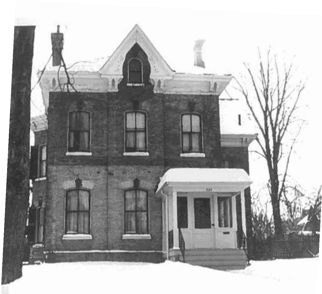
Image 3: View of front (north) façade of dwelling showing past entrance enclosure and steps; note discoloration line indicating possible previous porch extending across the façade (precise date of photo unknown; before 1990)
