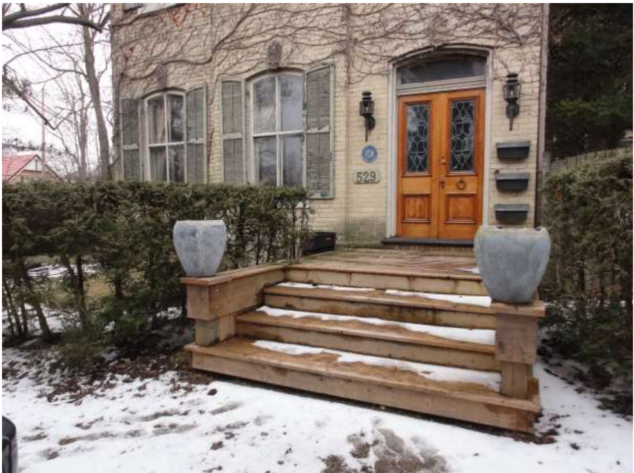
Image 2: View of non-conforming front entrance steps temporarily constructed
