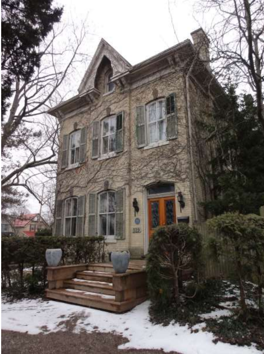
Image 1: View of front (north) façade of dwelling located at 529 Princess Avenue
