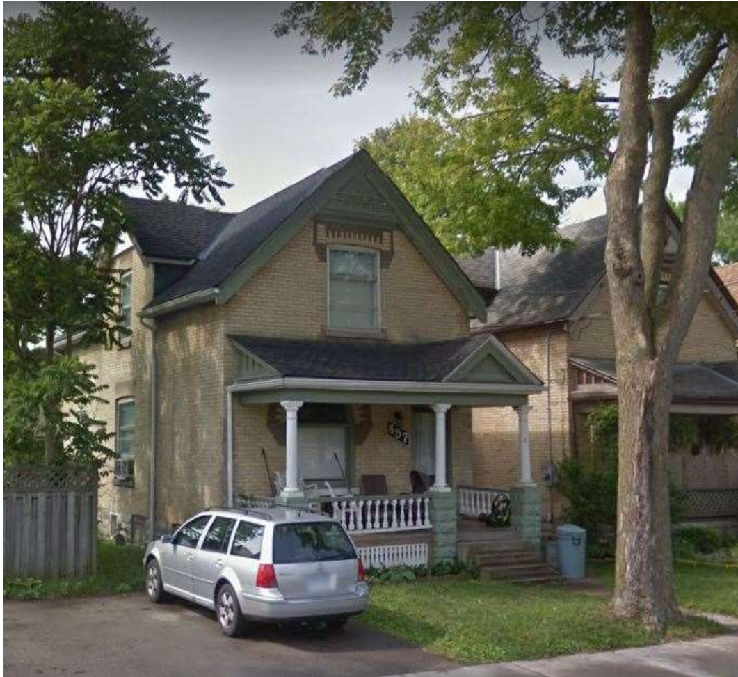
Image 5: View of the property located at 857 Princess Avenue – same typology with round columns and original spindles (April 6, 2018)
