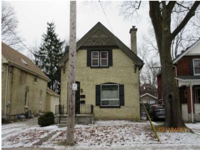
Image 2: View showing north (main) façade of the building located at 33 Beaconsfield Avenue prior to alteration (February 10, 2017).
