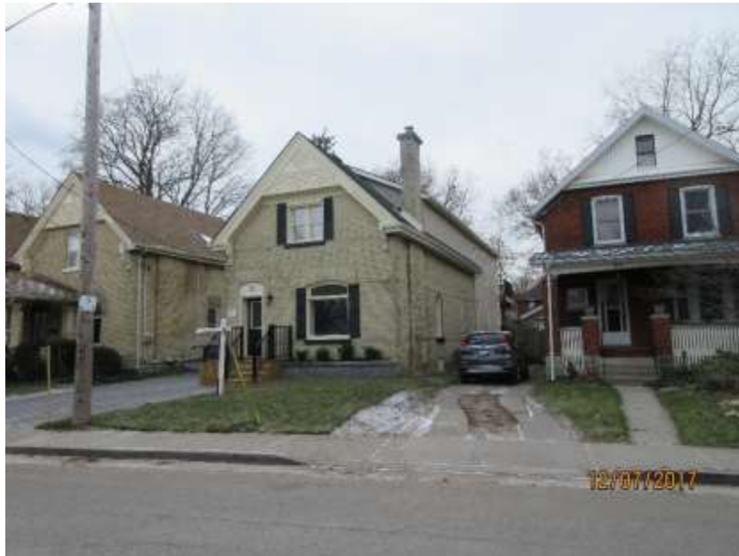
Image 7: View of the north (main) and west façades of the building located at 33 Beaconsfield Avenue subsequent to alteration (December 7, 2017). Note the enclosure of the window on the west façade, which has been filled with vinyl siding.
