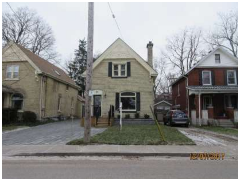
Image 6: View of the north (main) façade of the building located at 33 Beaconsfield Avenue subsequent to alteration (December 7, 2017).
