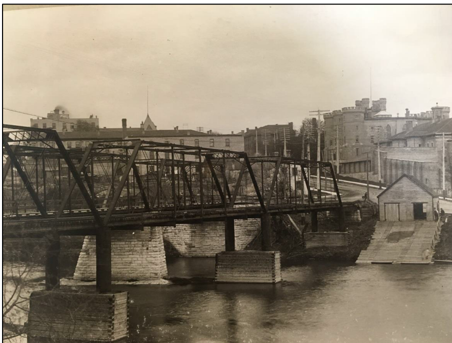
Image 10: Historic view from west side of the Thames River showing second Kensington Bridge, built in 1883. A second structure was built immediately south of the bridge supported on timber cribs to carry the LSR over the river (Western Archives. Western University. Regional Photograph Collection. RC 60221.)
