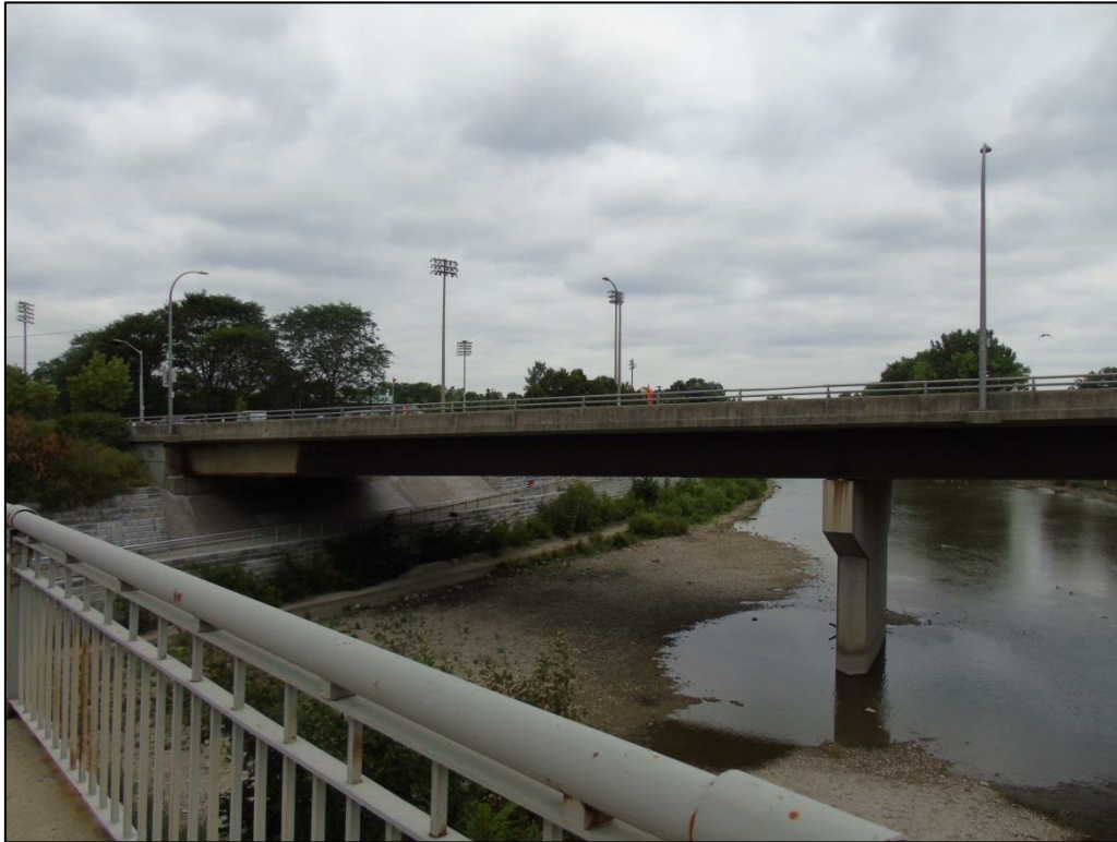
Image 2: View looking north showing the North Branch of the Thames River, as well as The Queen's Bridge located immediately to the north
