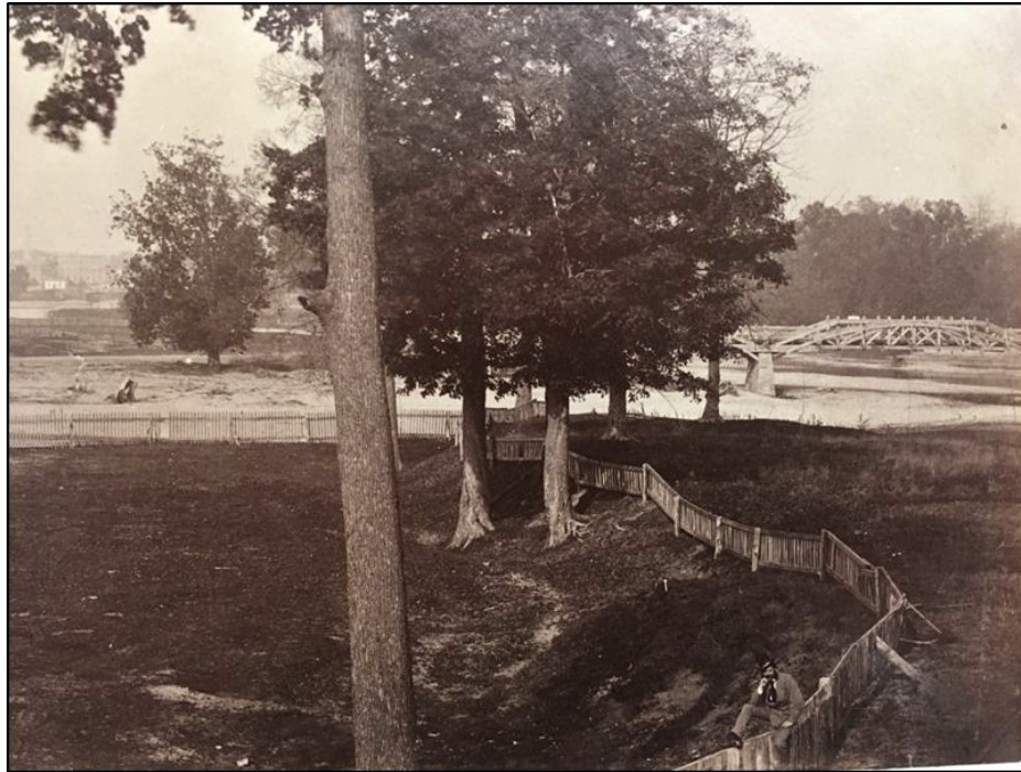
Image 7: Historic view showing 1871 Kensington Bridge at right. The bridge was a two-span timber frame structure over the river (Western Archives. Western University. Regional Photograph Collection. RC60186.)
