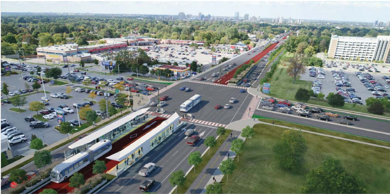
Wellington Road at Commissioners Road (looking north)
