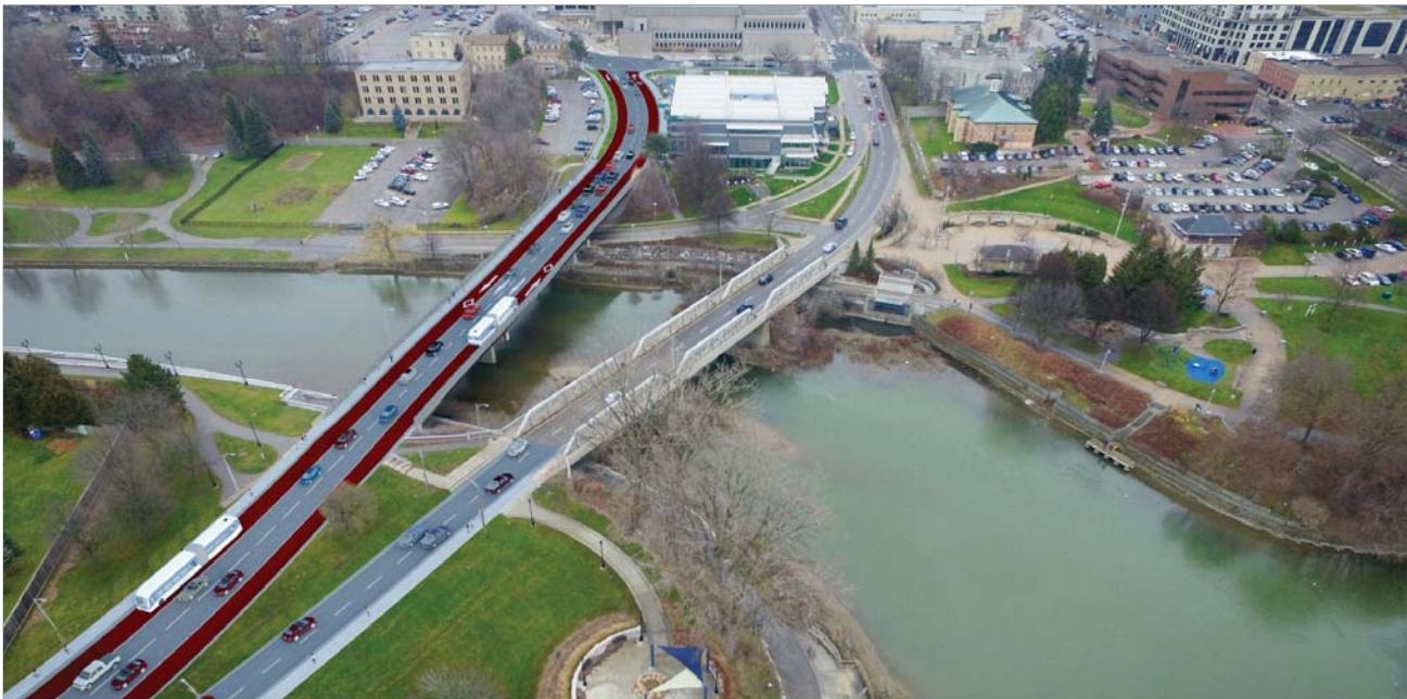
Riverside Drive across Thames River
