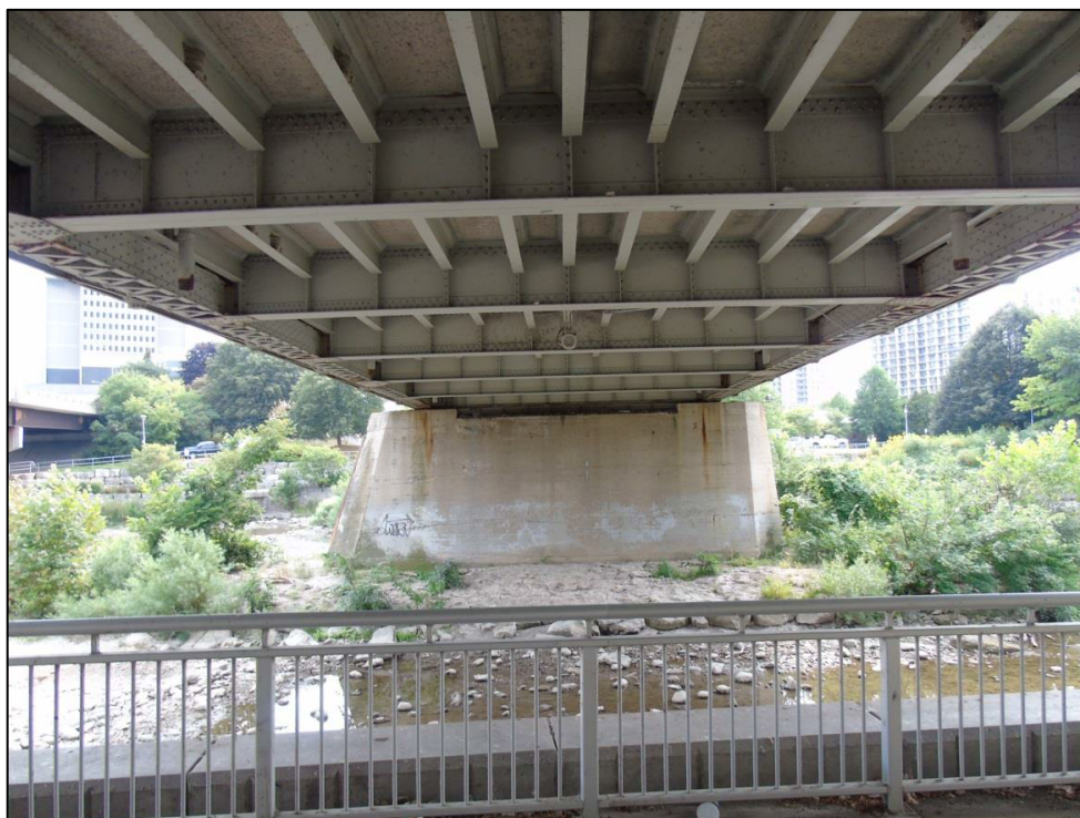
Image 27: View from east abutment looking towards west pier
