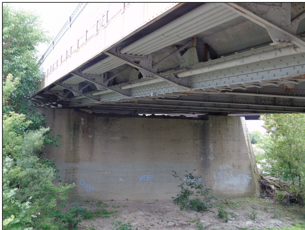
Image 25: East concrete pier located within the river
