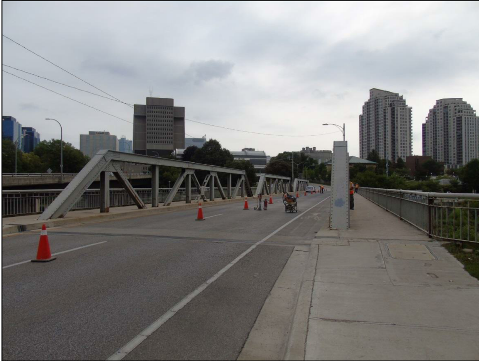
Image 38: View looking east showing deck and sidewalks
