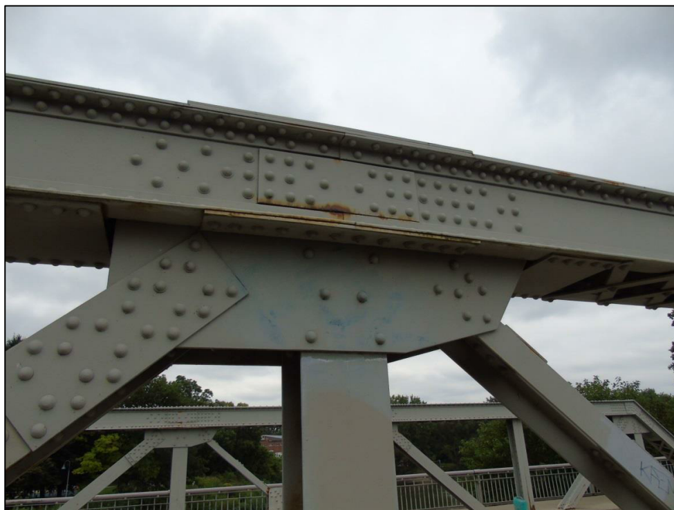
Image 29: Riveted connection of top chord showing gusset plates
