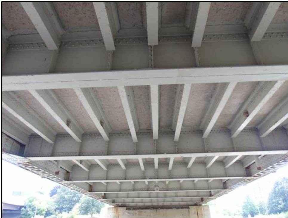
Image 35: View showing riveted steel beams and stringers along with concrete deck
