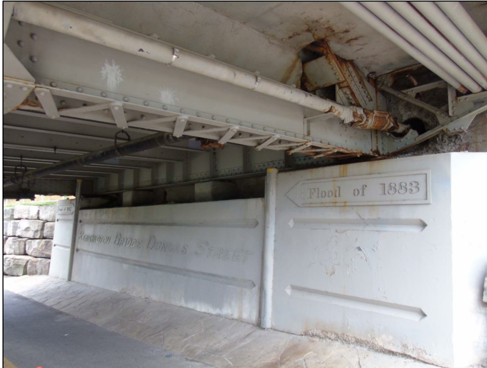
Image 22: View showing east abutment with "Flood of 1883" markers
