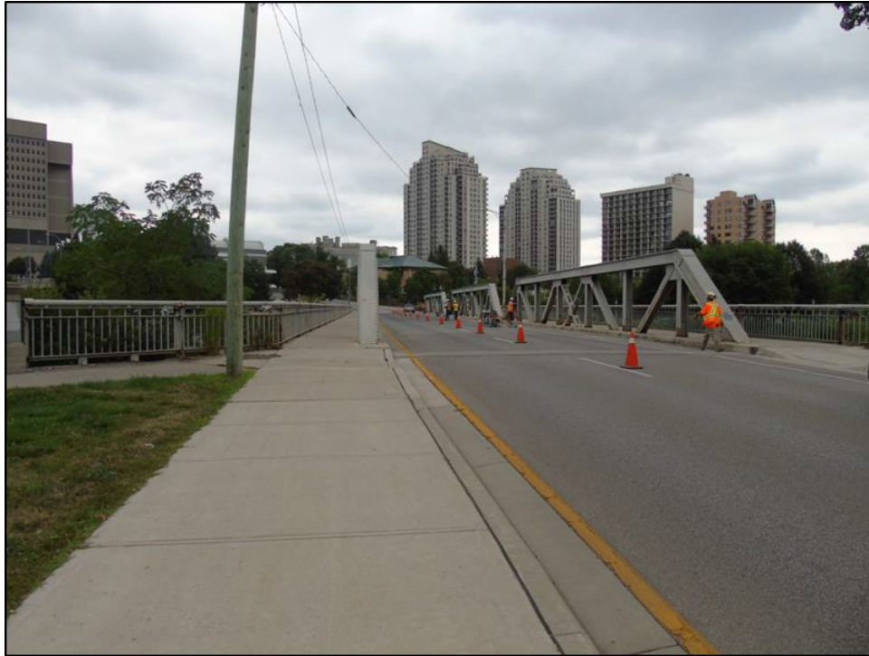
Image 20: View looking east showing west approach to the bridge
