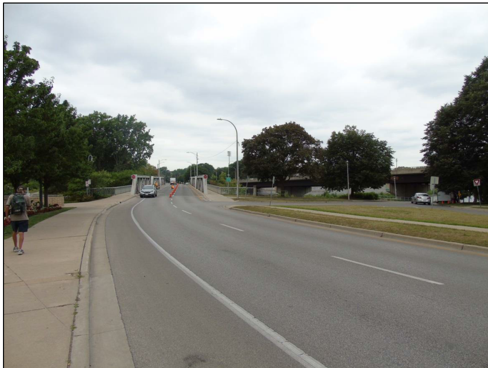
Image 21: View looking west showing east approach and curvature of the road
