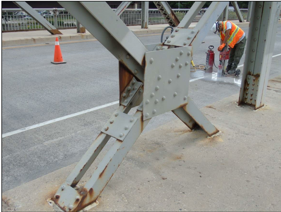
Image 34: View showing centre panel in the Warren truss
