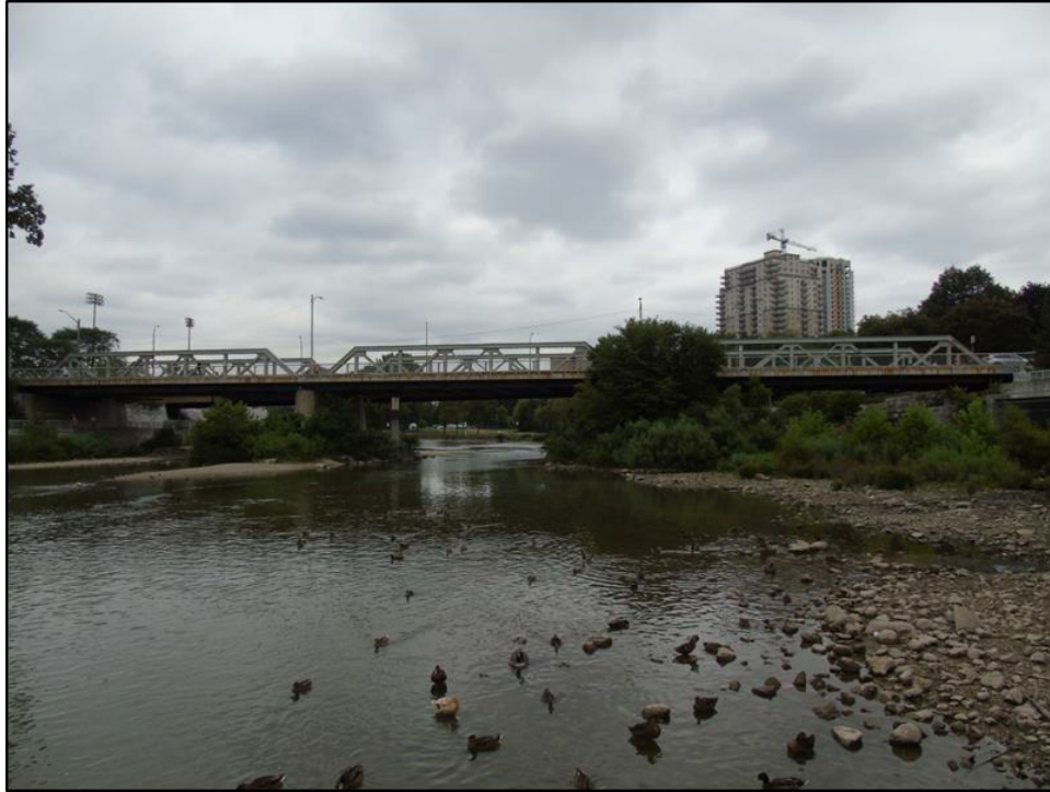
Image 13: View looking north showing three span Kensington Bridge structure over the Thames River
