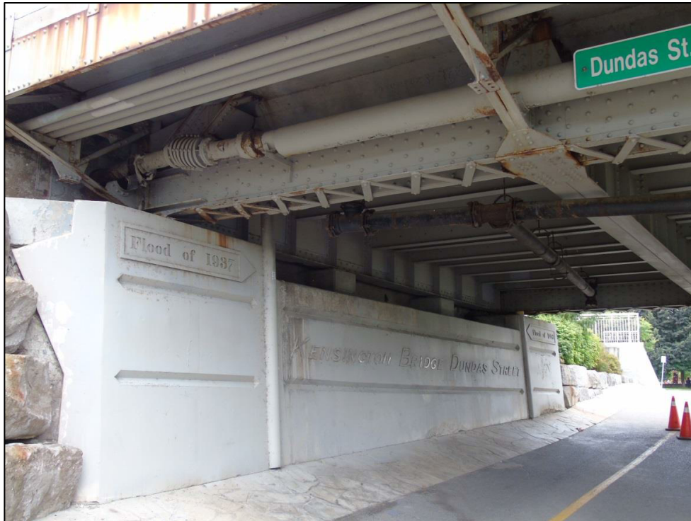
Image 24: North side of east abutment showing "Flood of 1937" marker
