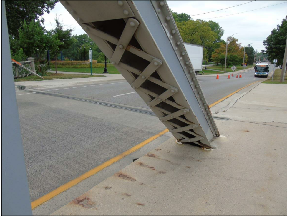
Image 30: View showing diagonal end post and riveted lattice
