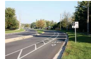
Buffered bicycle lane in London.
