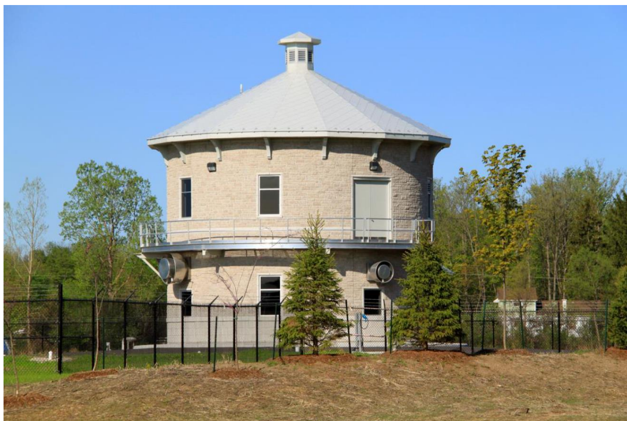
Figure 1 – Wonderland Pumping Station
