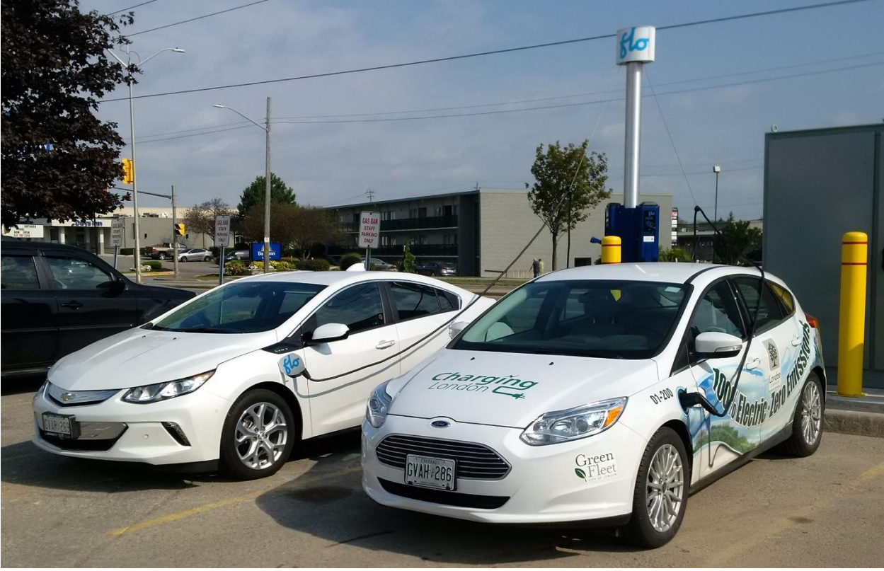
Figure 3 - FLO Charging Station at Canadian Tire on Wellington Road South
