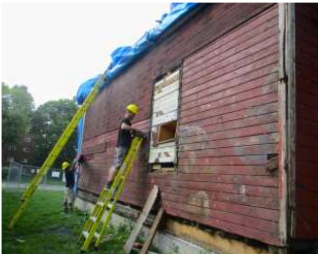
Exposing the original wide tongue-and-groove planks of the east wall
