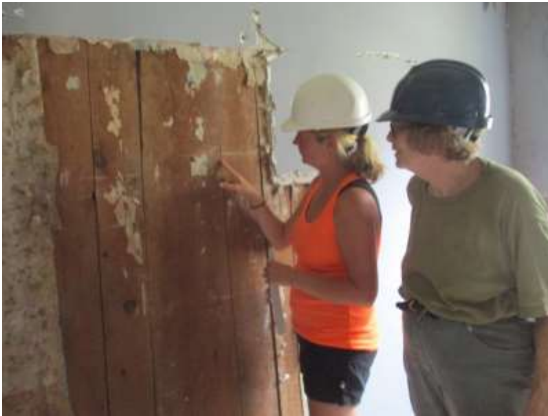
Hilary Neary and Tara Jenkins stripping wallpaper from vertical planks between two rooms in the western portion of the house
