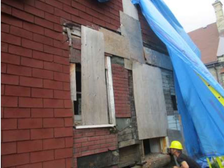
Varieties of materials covering the rear (north) wall
