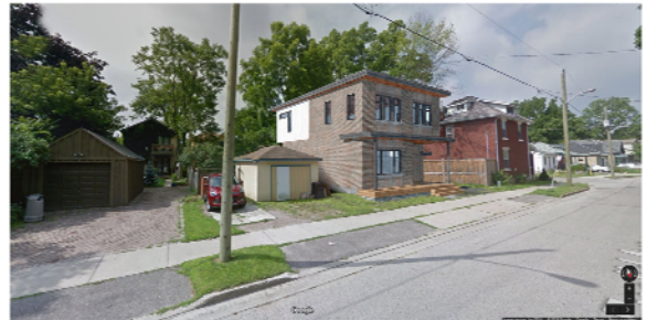
Front elevation showing proposed building at 67 Euclid Avenue with its front façade in alignment with the abutting property at 2 Birch Street
