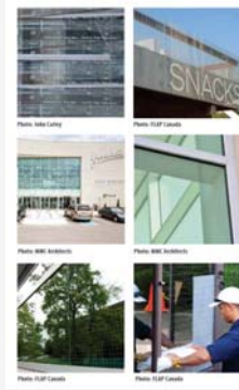
Effective glass treatments for bird-friendly building design. Photographs from Toronto Bird-Friendly Best Practices Glass ©
