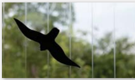
A window with visual marker strips and a bird used to prevent bird strikes. Photograph from www.smith.edu/news/preventing-bird-collisions-at-mccorrell/
