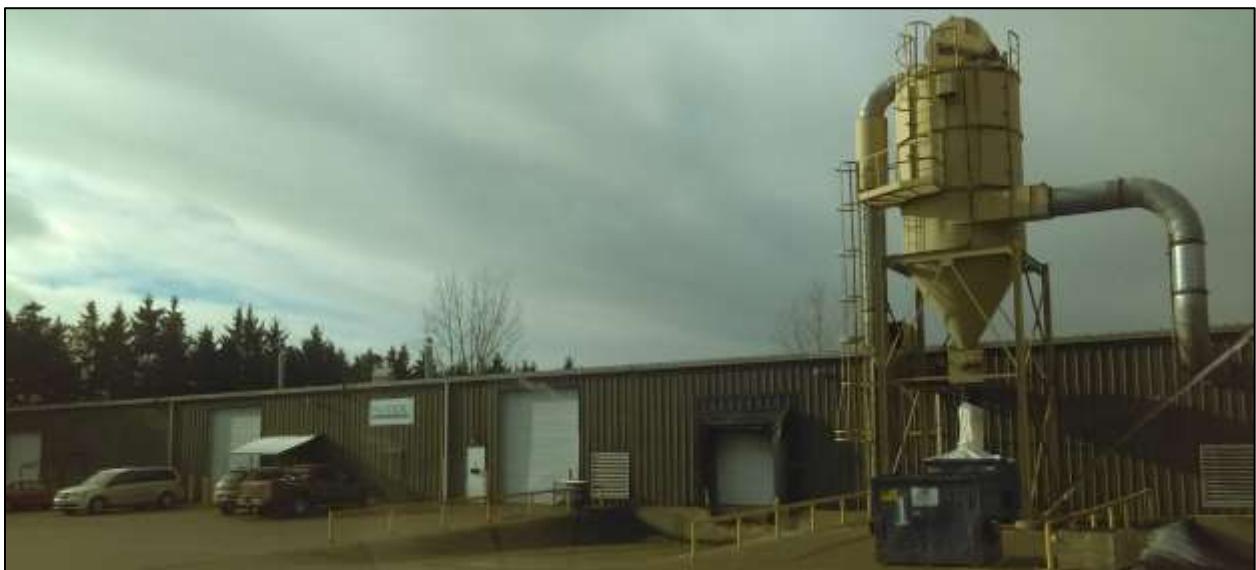
Figure 2: Subject Site – Rear Building Photo
