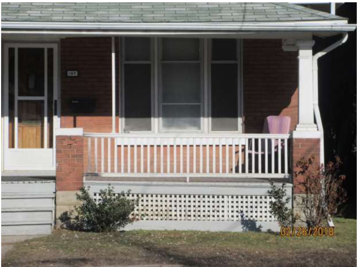
Image 8: Detail of porch balustrade at appropriate height with appropriate details and finish located at the building at 197 Wharnccliffe Road North. Note the height of the balustrade is at the appropriate height to match the capstone of the brick plinths.
