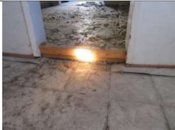
Image 10: Detail of juncture between main house and kitchen wing (2015-12-11).
