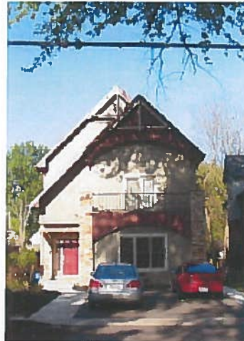
599 Maitland Ave. – New infill matches the scale of adjacent buildings but permits front yard parking. Parking should be located in the rear or side yard when possible.
