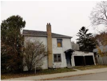
69 Wilson Avenue, south elevation facing Rogers Avenue
