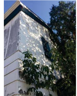
69 Wilson Avenue, view of corner cladding detail
