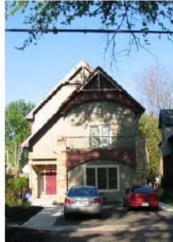
599 Maitland Ave. – New infill matches the scale of adjacent buildings but permits front yard parking. Parking should be located in the rear or side yard when possible.
