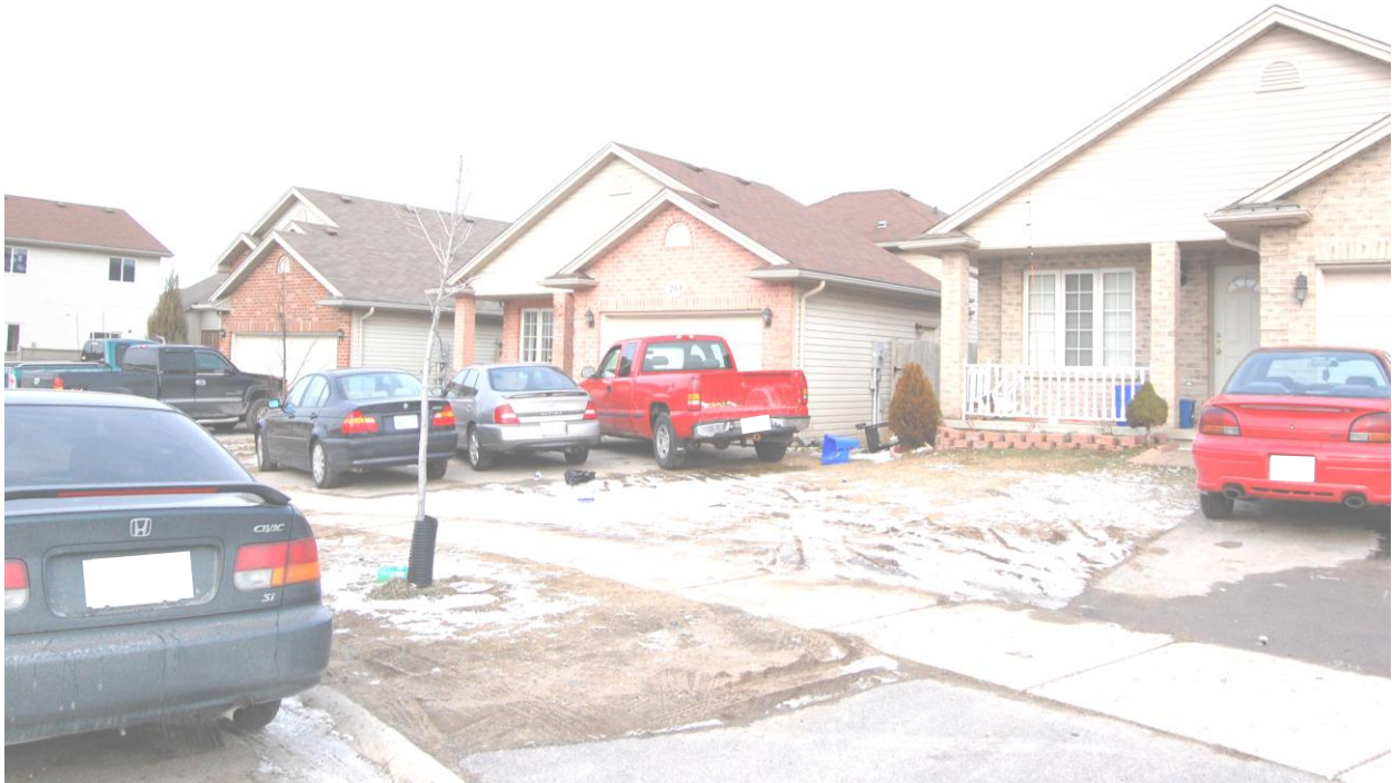
Photo illustrating the property damage caused when vehicles traverse the landscaped open space in an effort to park vehicles parallel to the street
