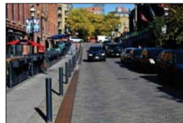
Example Detectible Warning Surface – Market Street Toronto
