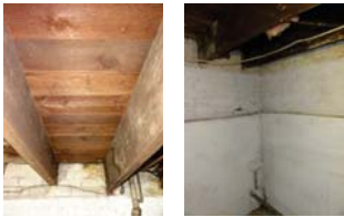
View of floor joists from basement – Brick exterior basement wall
