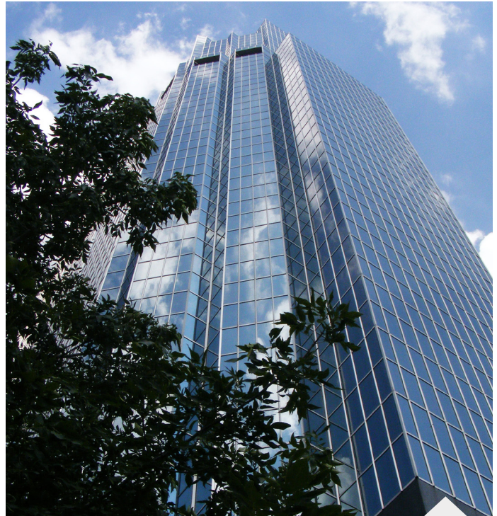
One London Place provides 382,000 square feet of leasable office space downtown.
