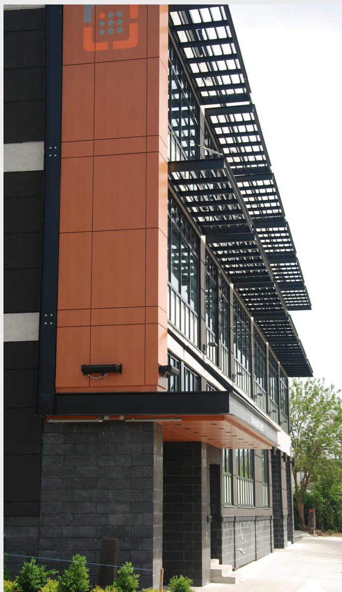
The Cube underwent extensive renovations in 2015 to house Arcane Digital.
