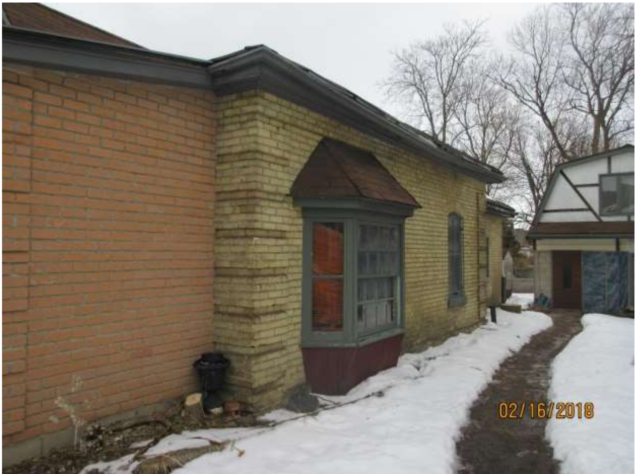
Image 4: View of west façade of building showing front addition, original structure, and rear addition of the building located at 504 English Street, and detached out building.
