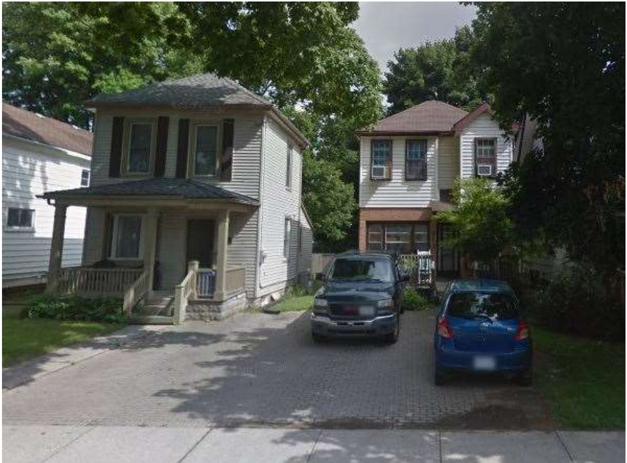
Image 5: View of (north) façades of the buildings located at 64 and 66 Euclid Avenue
