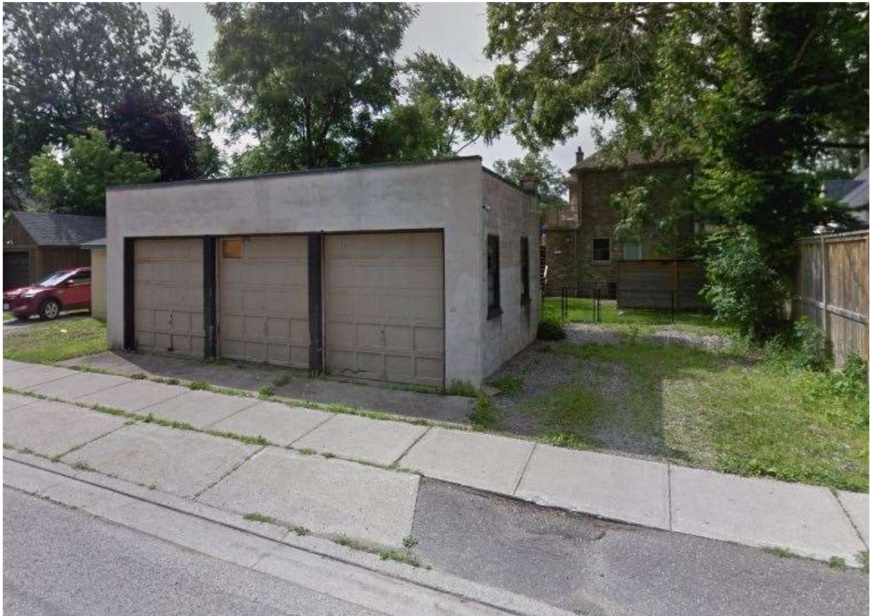
Image 1: View of front (south) façade of the existing detached garage located at 67 Euclid Avenue.
