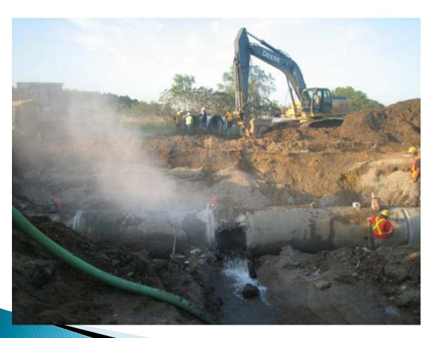
Spent part of the day shutting down the section, pumping off the field, and building a temporary access road to limit the damage to crops.
