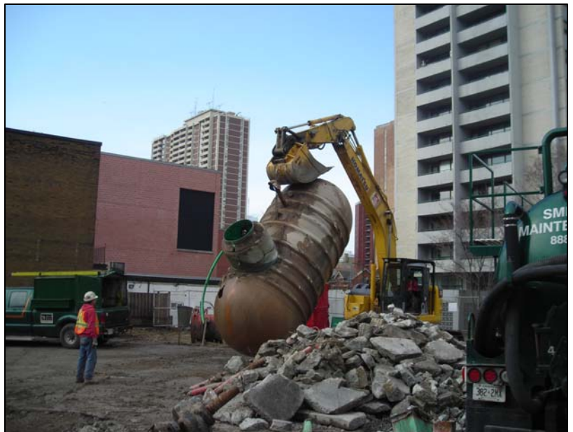
Removal of underground storage tank.
