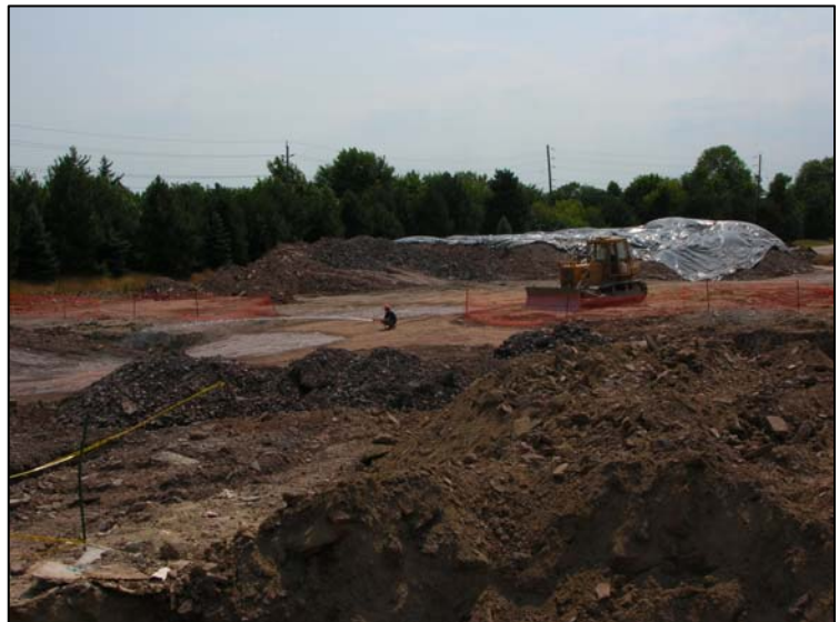
On-site remediation activities.
