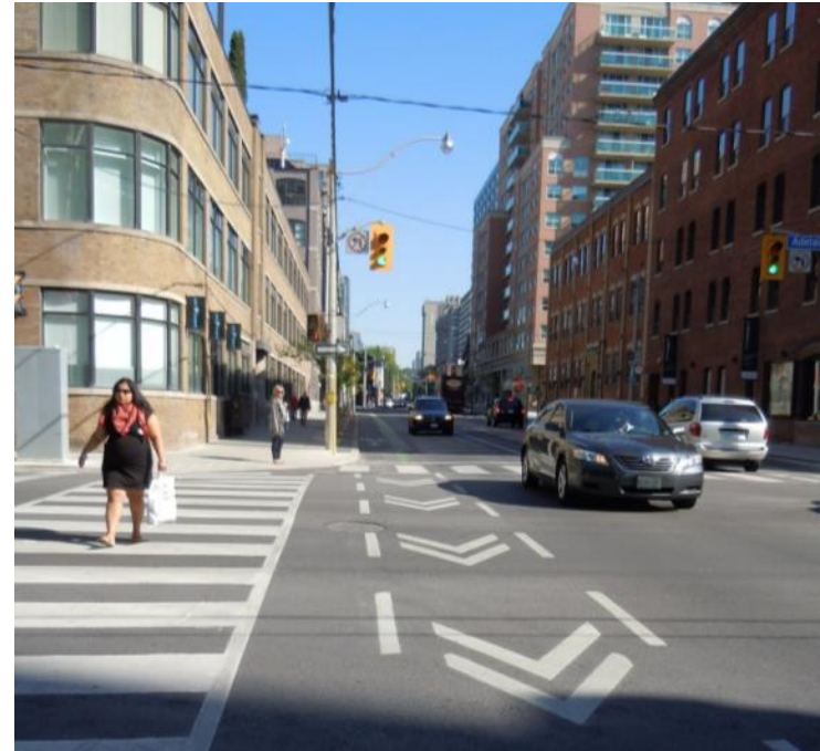
Off-set Intersection: Chevrons are used to mark the facility through the intersection.
