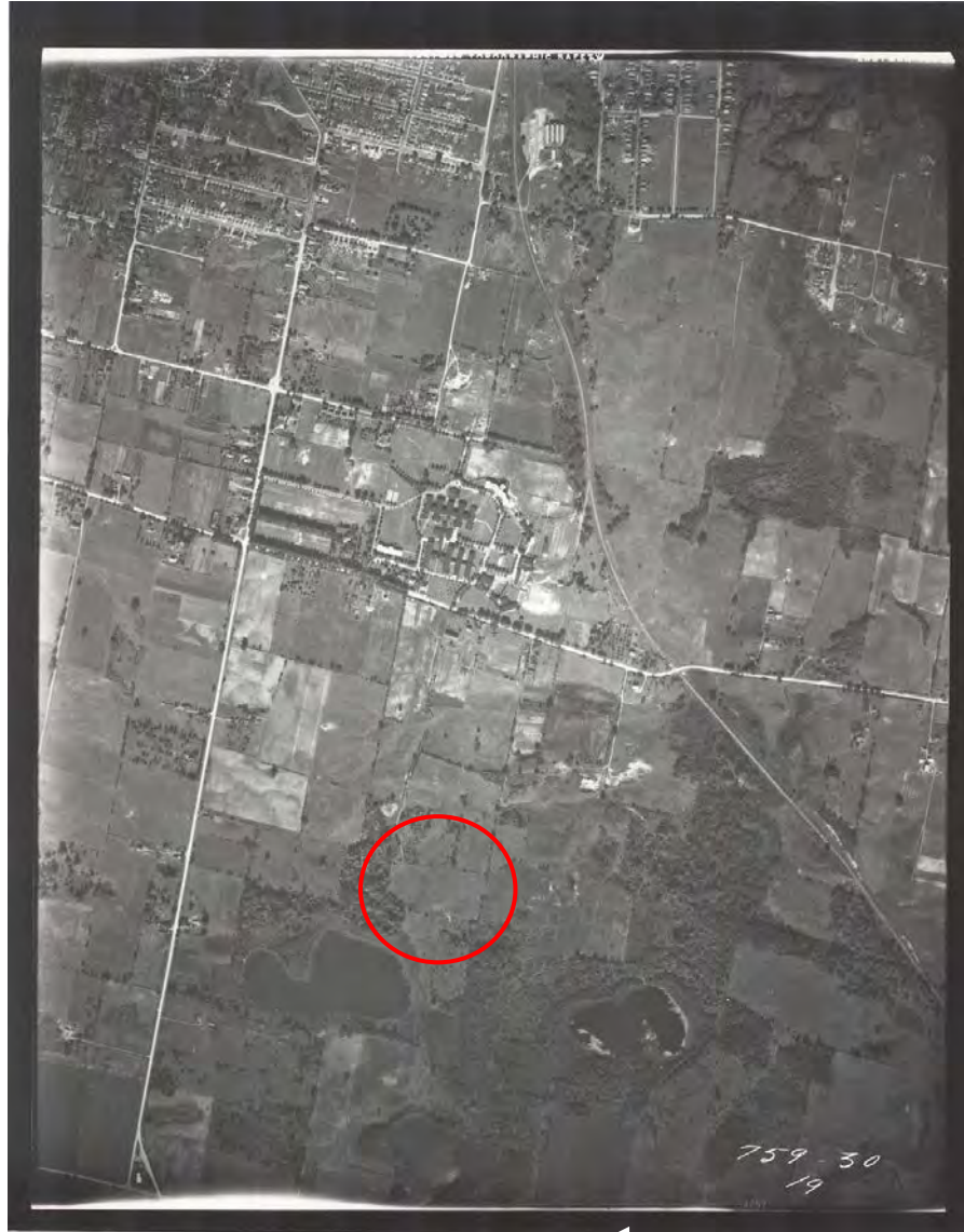
Figure 3: 1942 Aerial Photograph of study area, Map and Data Centre, University of Western Ontario (circle denotes site of future Western Counties Centre)
