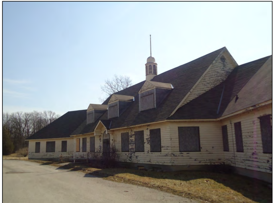
Figure 16: Rear view of the former Wellington Pavilion, 2012.
