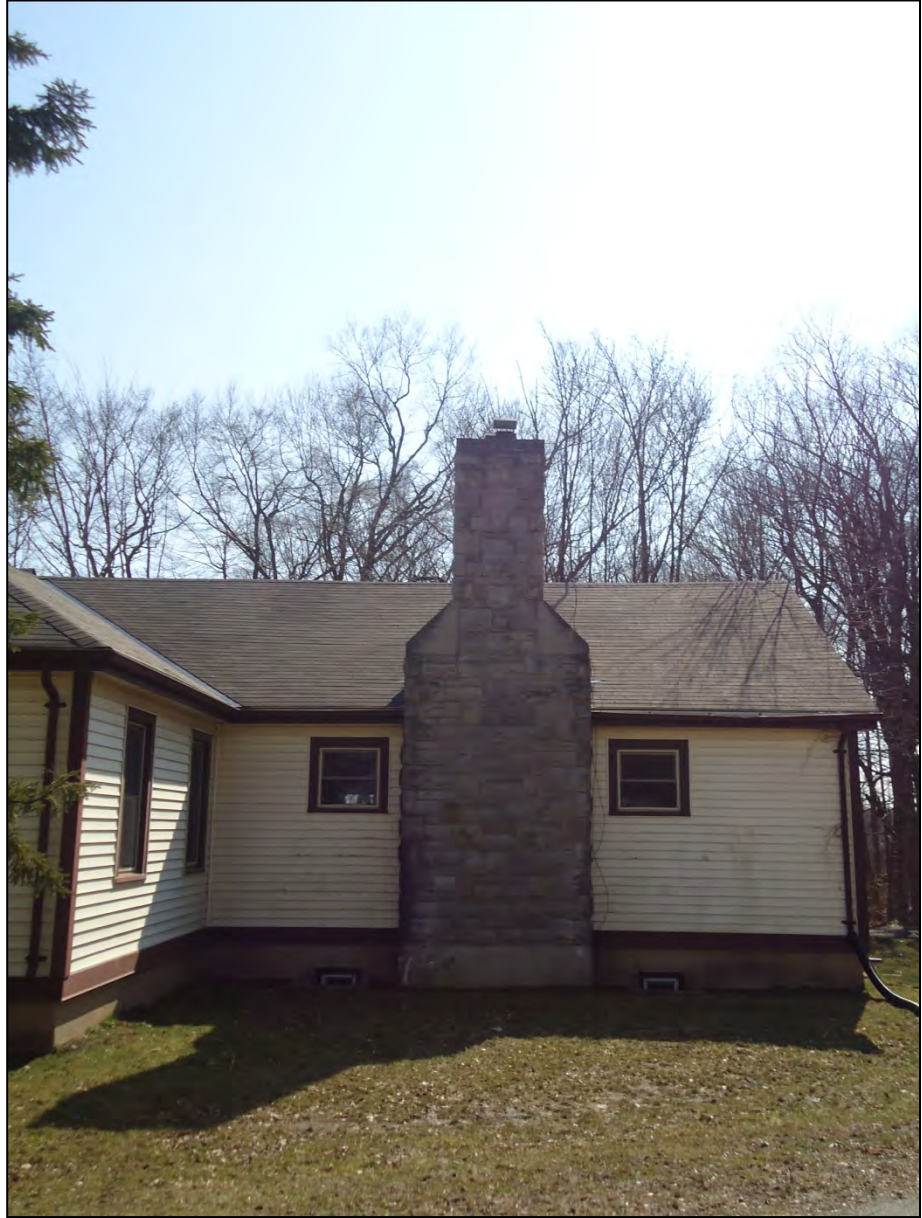
Figure 12: Rear view featuring chimney, 2012.
