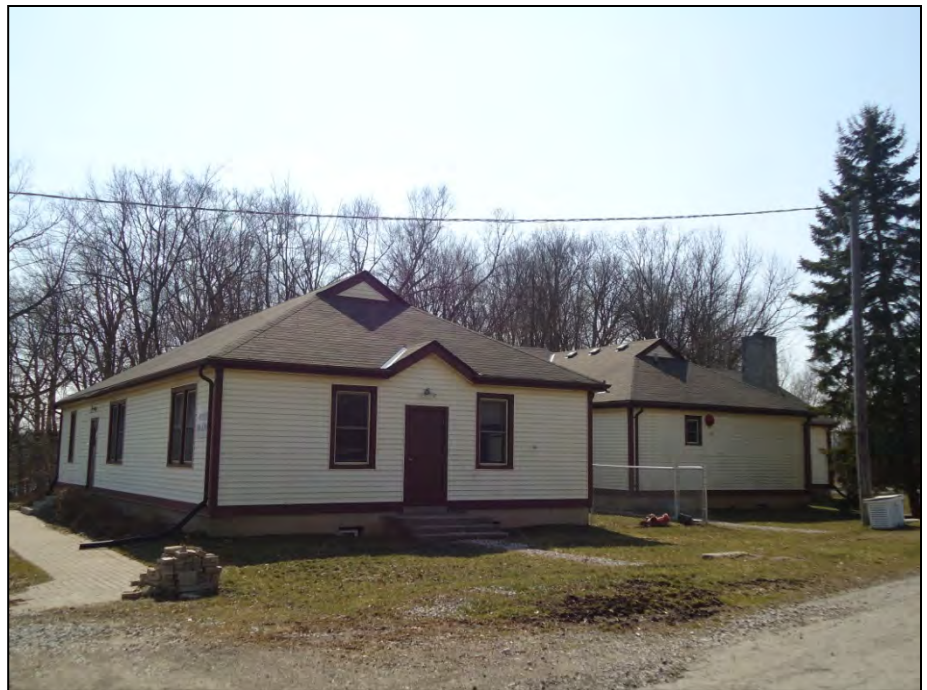
Figure 11: Rear view of existing cottage pavilion, 2012.
