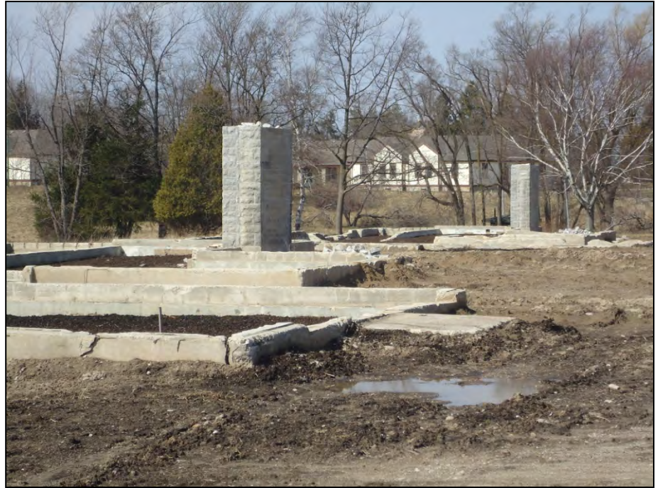
Figure 18: View of foundation ruins and chimneys looking toward remaining cottage, 2012.
