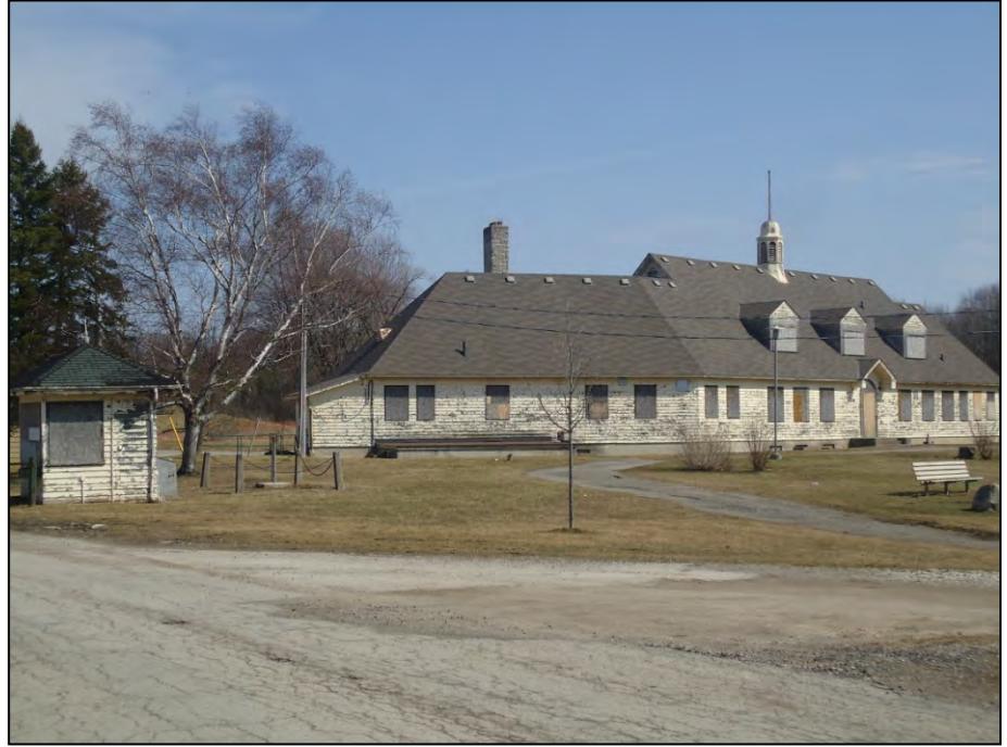
Figure 15: View of front and side wing of former Wellington Pavilion, with gatehouse to left, 2012.
