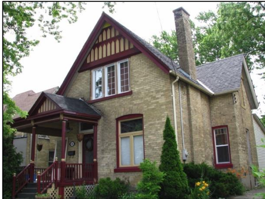
Figure 5. 98 Stanley Street adjacent to east of 100 Stanley Street.
