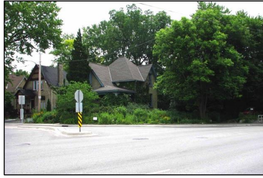
Figure 4. View southeast to 100 Stanley Street with 98 Stanley Street in the background.
