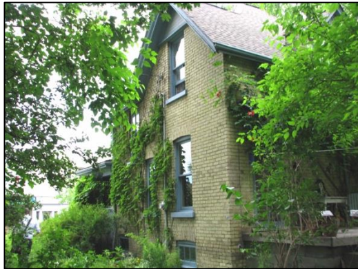
Figure 17. View northeast to west elevation.
