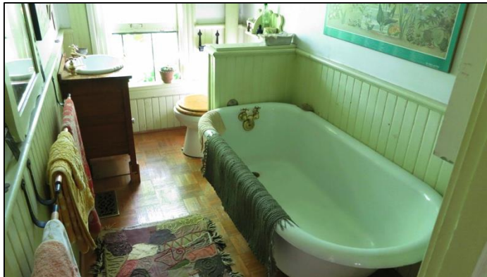
Figure 39. Wainscoting in the bathroom, second floor.
