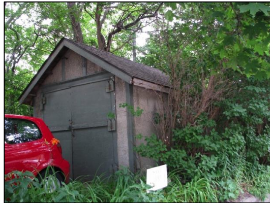
Figure 8. Garage located on the southwest corner adjacent to Wharncliffe Road South.
