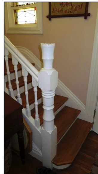
Figure 27. Newel post on main staircase, ground floor.
