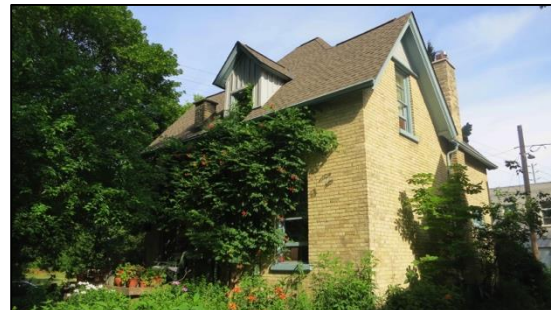
Figure 14. Southeast corner of the house.
