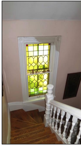
Figure 37. Window on west wall, on staircase landing.
