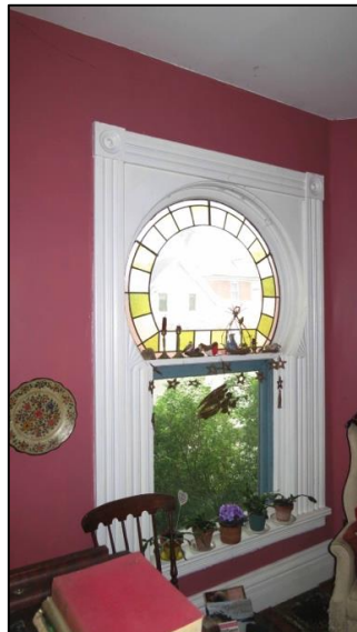
Figure 32. Wood trim around the key hole window in living room, ground floor.
