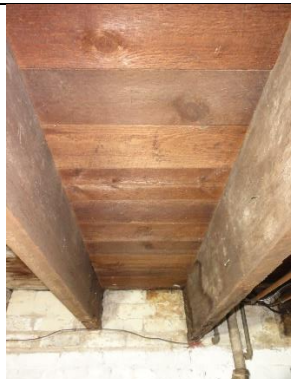
Image 11: View of floor joists from basement
