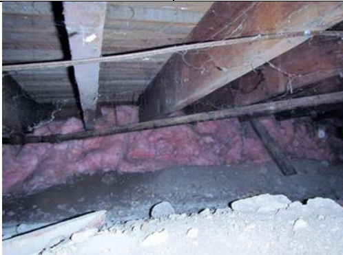
Image 13: View of crawl space beneath rear portion of cottage
