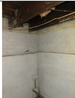
Image 12: Brick exterior basement wall
