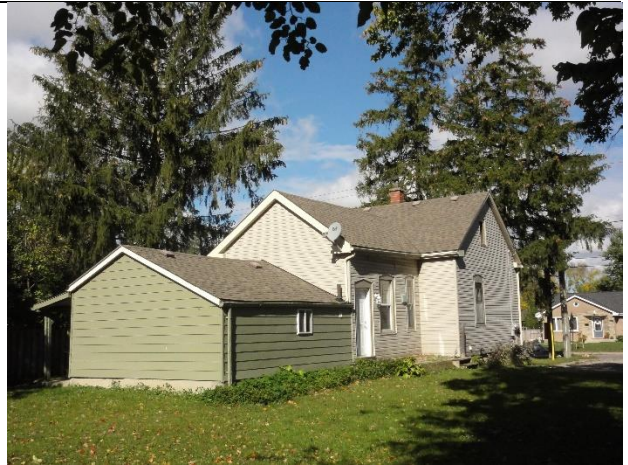
Image 8: Rear elevation showing addition
