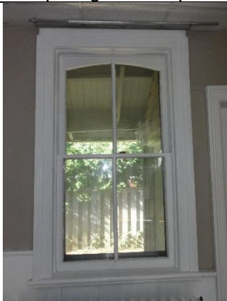
Image 9: Interior view of original windows
