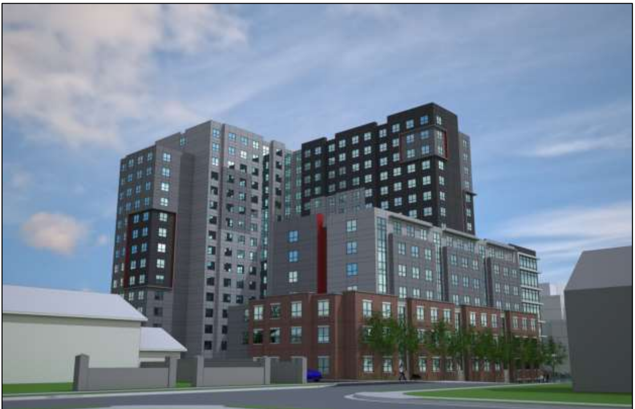
Final Design (August, 2017) – 3-storey base along Talbot, stepback to 7-storeys, 16-storeys of height has been moved to the rear and north side of the property.
