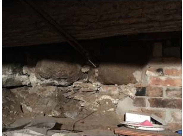
Image 10: Rubble stone and masonry interior supporting foundation wall
