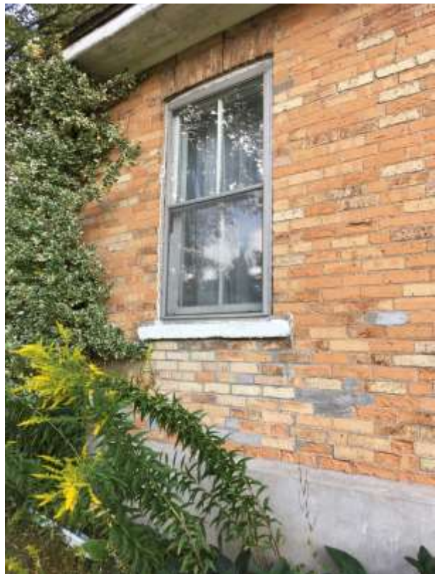
Image 15: Partial west elevation showing re-bricked work beneath window
