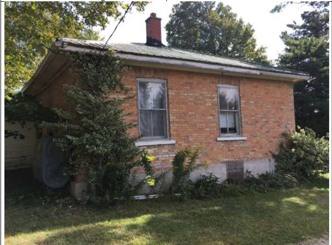
Image 21: South-east corner detail view showing new brickwork in differing tone and detailing
