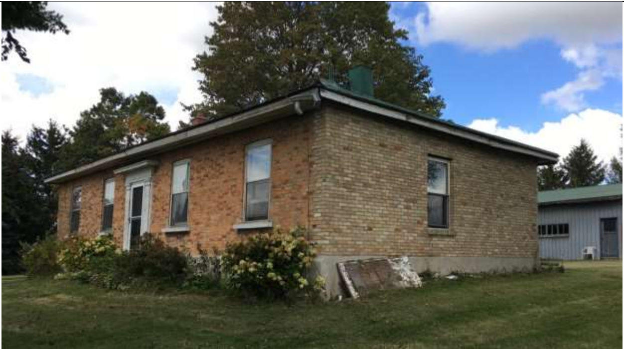
Image 20: South-east corner view showing new brickwork in differing tone and detailing – full east elevation
