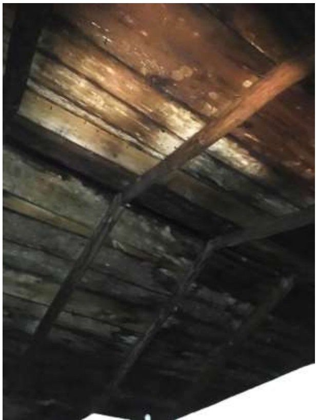
Image 13: Roof framing at ridge
