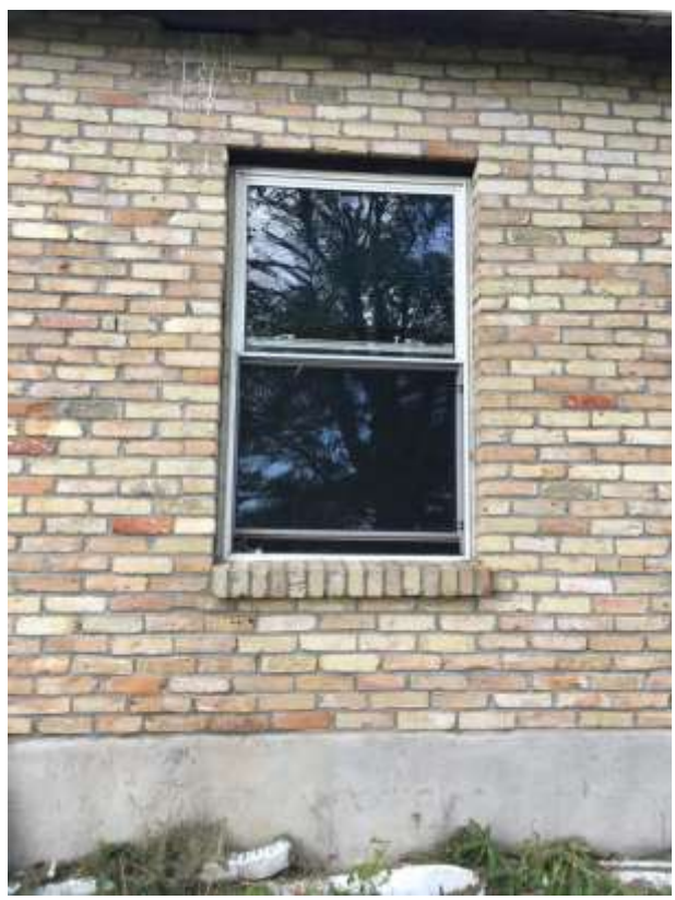
Image 18: South-east façade showing new brickwork in differing tone and detailing
