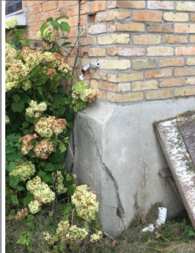
Image 21: South-east corner detail view showing new brickwork in differing tone and detailing
