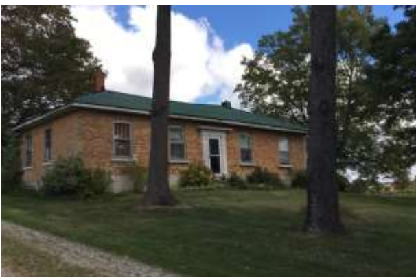
Image 16: South-west corner view; front elevation of cottage
