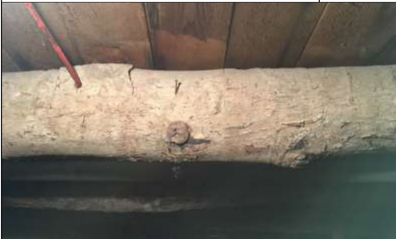
Image 9: Rubble stone outer foundation wall with "dressed" timber log framing
