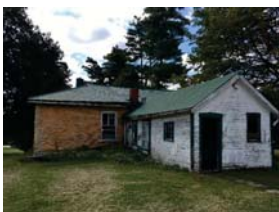
Frame addition at rear with wood clapboards, windows and trim
