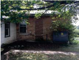
North (rear) elevation – partial, showing brick infill
