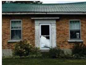
Front elevation and Neoclassical doorway surround
