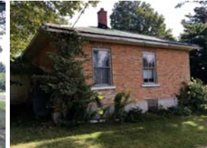
West elevation – showing brick infill beneath window
