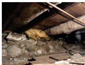
Rubble stone outer foundation wall with "dressed" timber log framing
