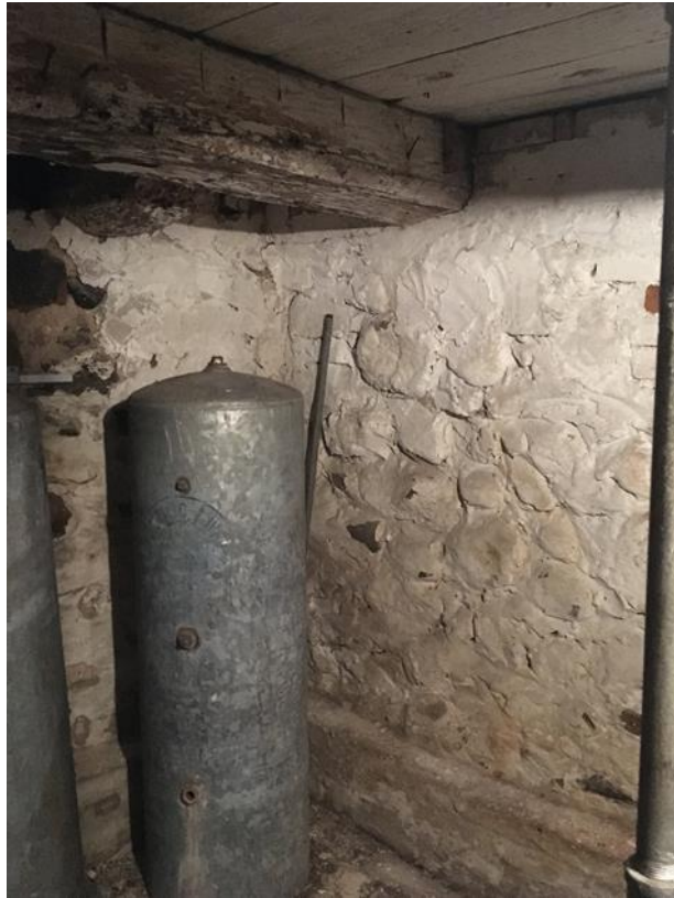
Image 12: Interior supporting basement wall – hand hewn framing with chamfered edges
