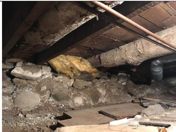
Image 9: Rubble stone outer foundation wall with "dressed" timber log framing
