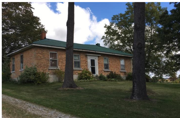
Image 16: South-west corner view; front elevation of cottage
