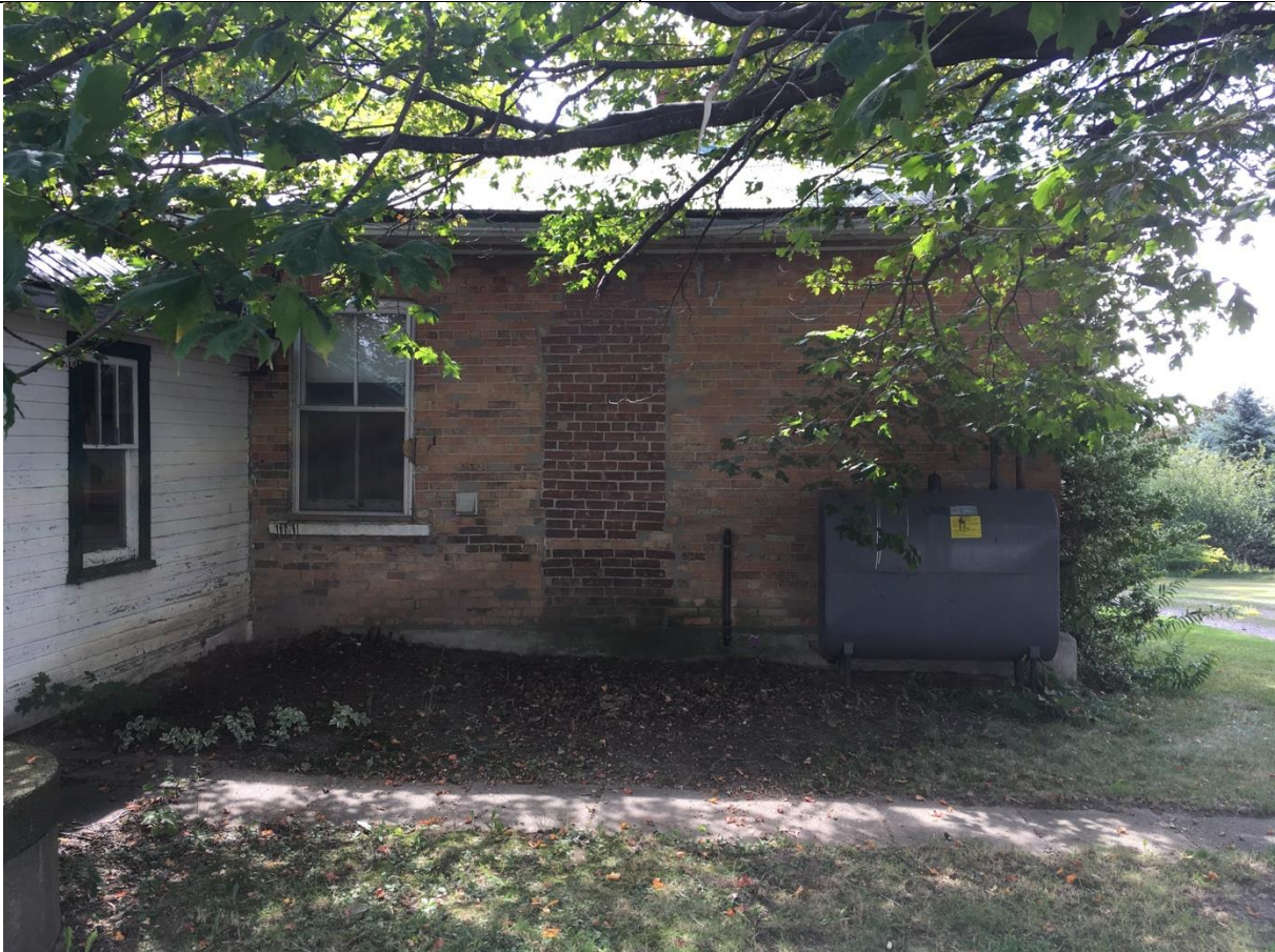
Image 19: North (rear) elevation – partial, showing wood frame addition
