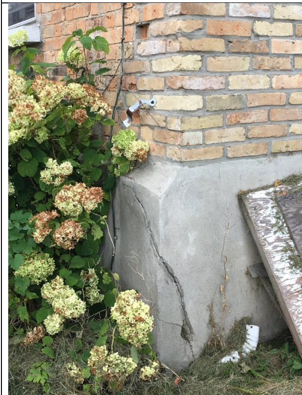
Image 21: South-east corner detail view showing new brickwork in differing tone and detailing
