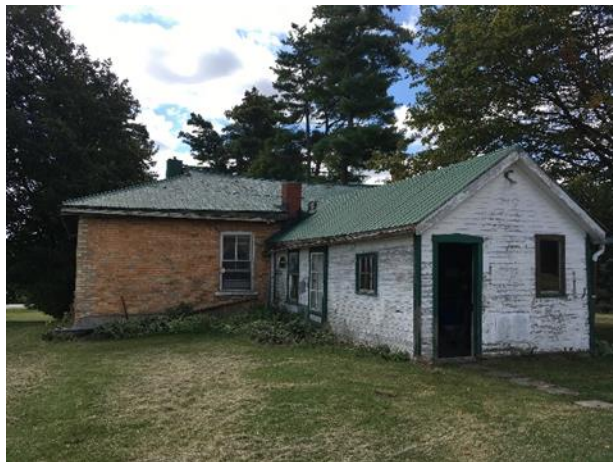
Image 14: Frame addition at rear with wood clapboards, windows and trim
