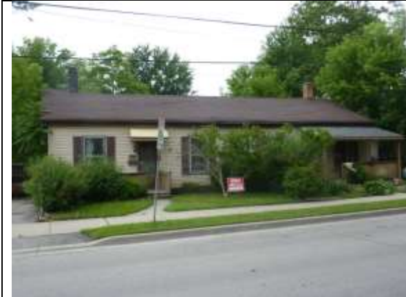
Image 1: Building formerly located at 471-473 Elizabeth Street, demolished in 2014 (June 24, 2014).
