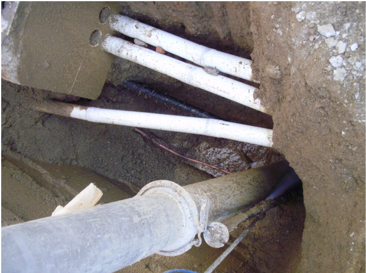
Figure 1 – Underground Utility Congestion
