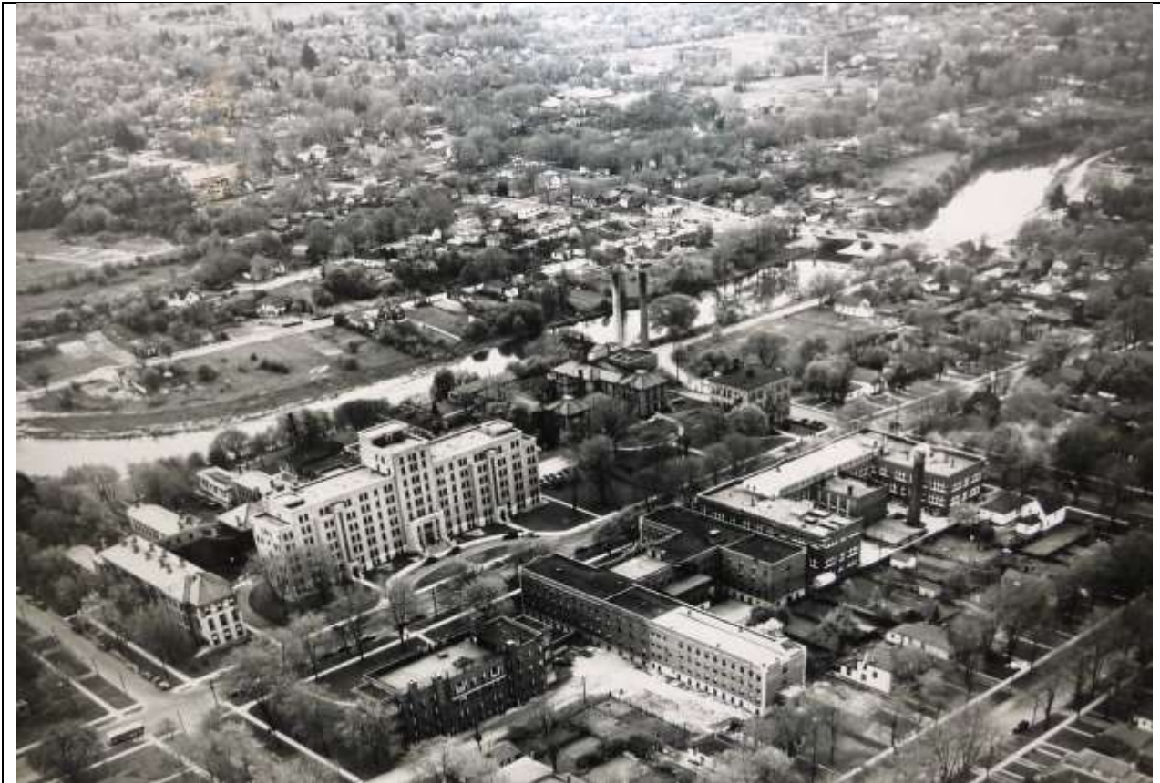
Image 10: Old Victoria Hospital Lands, aerial view c1930 – Colborne Building (to the left), 2011 (Tausky, p75)
