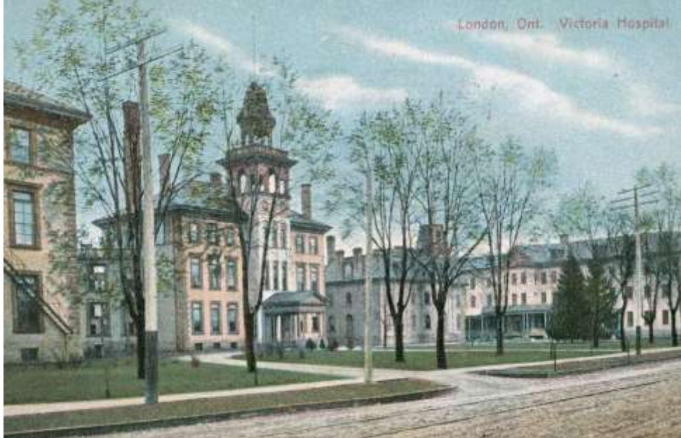
Image 4. Postcard based on tinted photograph of Victoria Hospital. Note sandstone window trim on the Colborne Building (to the left) (Tausky, p73)
