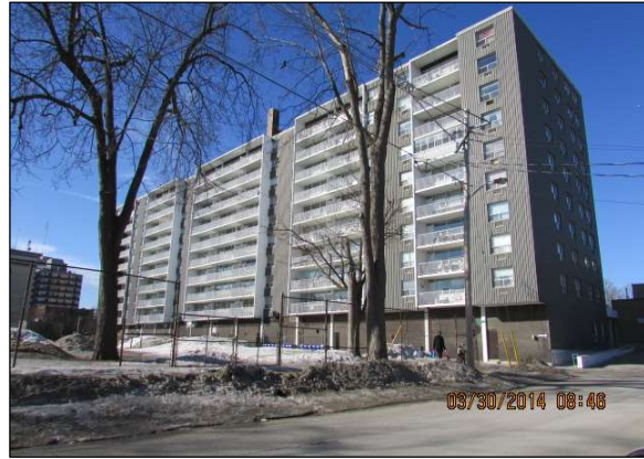
Wellington 520 Centennial House
