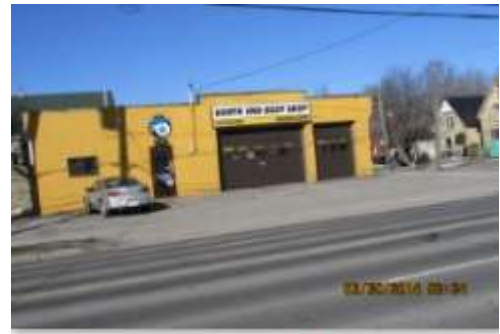
Adelaside 580 Industrial Autobody Shop
