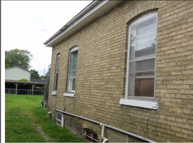
Image 3: Side elevation – west, showing existing window openings
