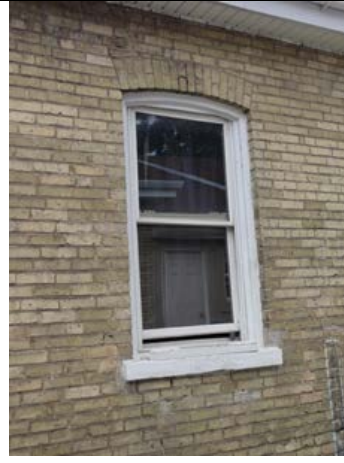
Image 4: Side elevation – east, showing existing window opening
